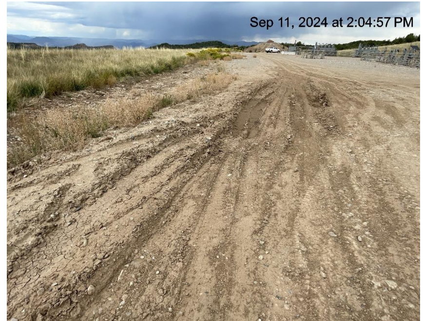
Photo # 9840 Lack of stabilization/compaction
