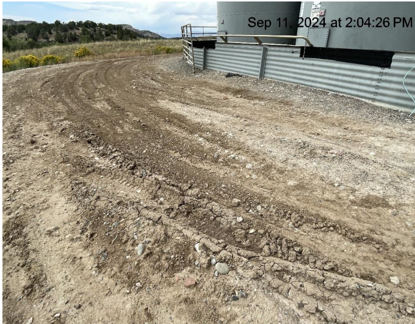
Photo # 9839 Lack of stabilization/compaction
