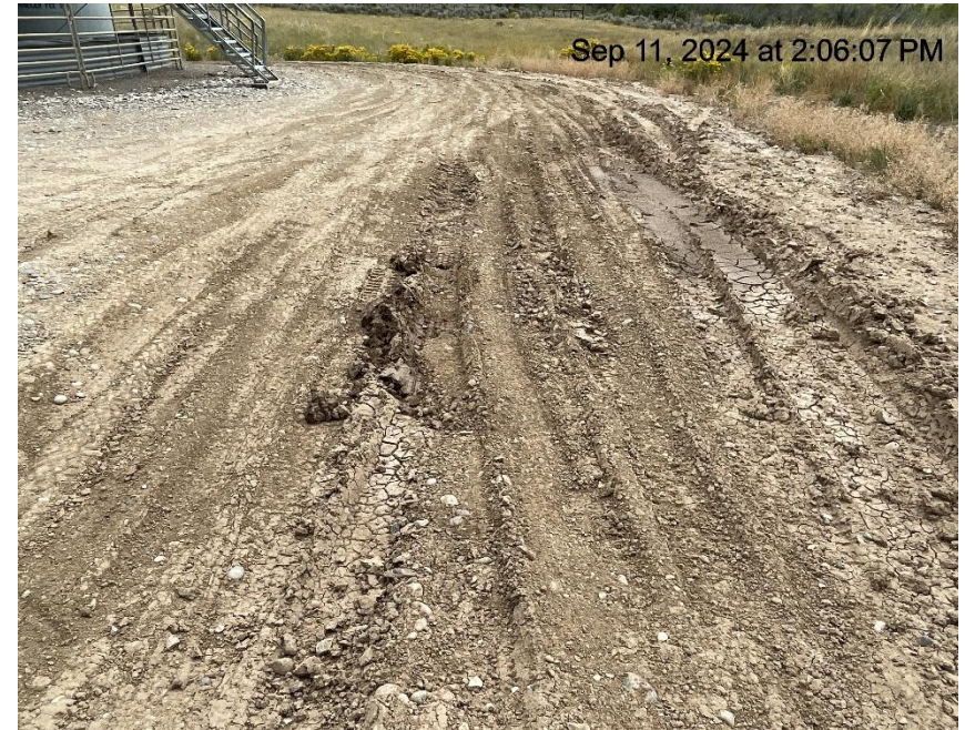
Photo # 9842 Lack of stabilization/compaction
