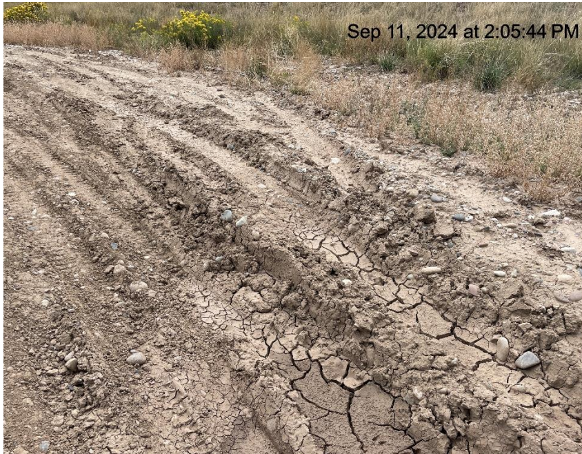
Photo # 9841 Lack of stabilization/compaction
