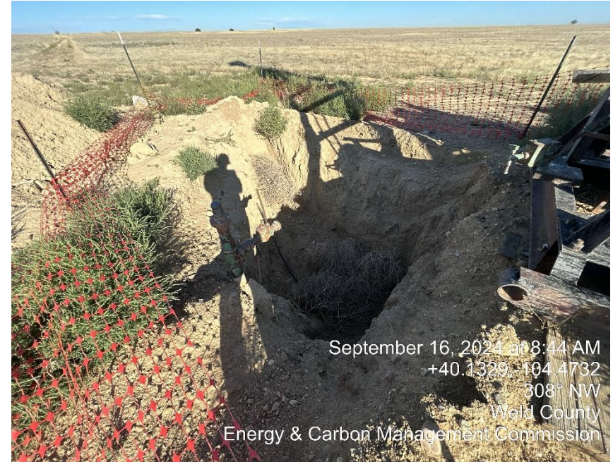
Safety Fence around the open hole needs to be repaired.
