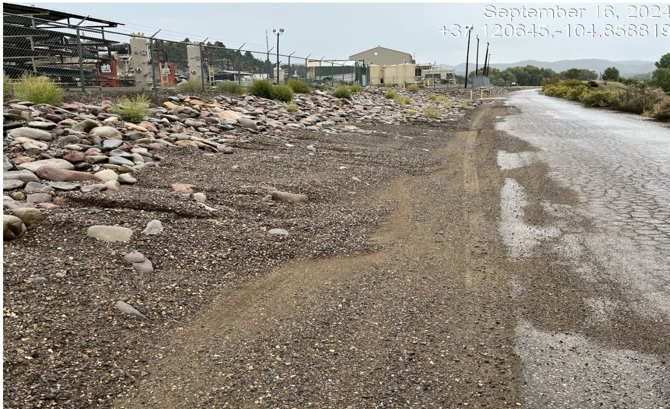
Photo 2. Facing northeast along the main paved road. The sediment and gravel along this area should be cleaned out to prevent sediment movement onto the paved road.
