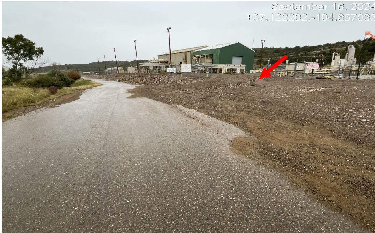
Photo 1. Facing southwest along the main road to the compressor facility. There is erosion occurring at the red arrow which is directing sediment onto the main road. Sediment needs to be removed from the paved road and sediment controlled.
