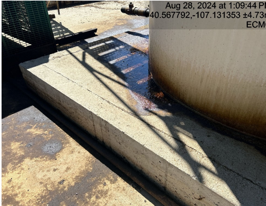
Possible tank leaking
