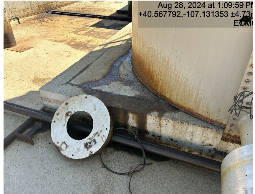
Possible tank leaking and burner assembly parts
