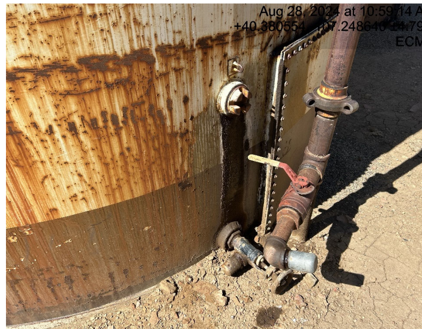
Tank plug leaking
