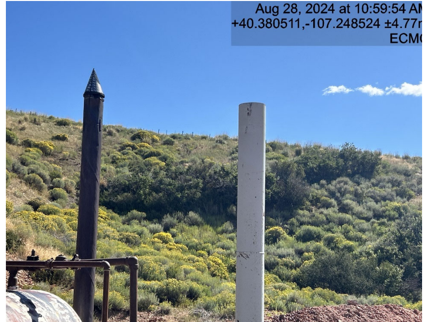
Separator has noticeable bird protector while heat treater is unknown
