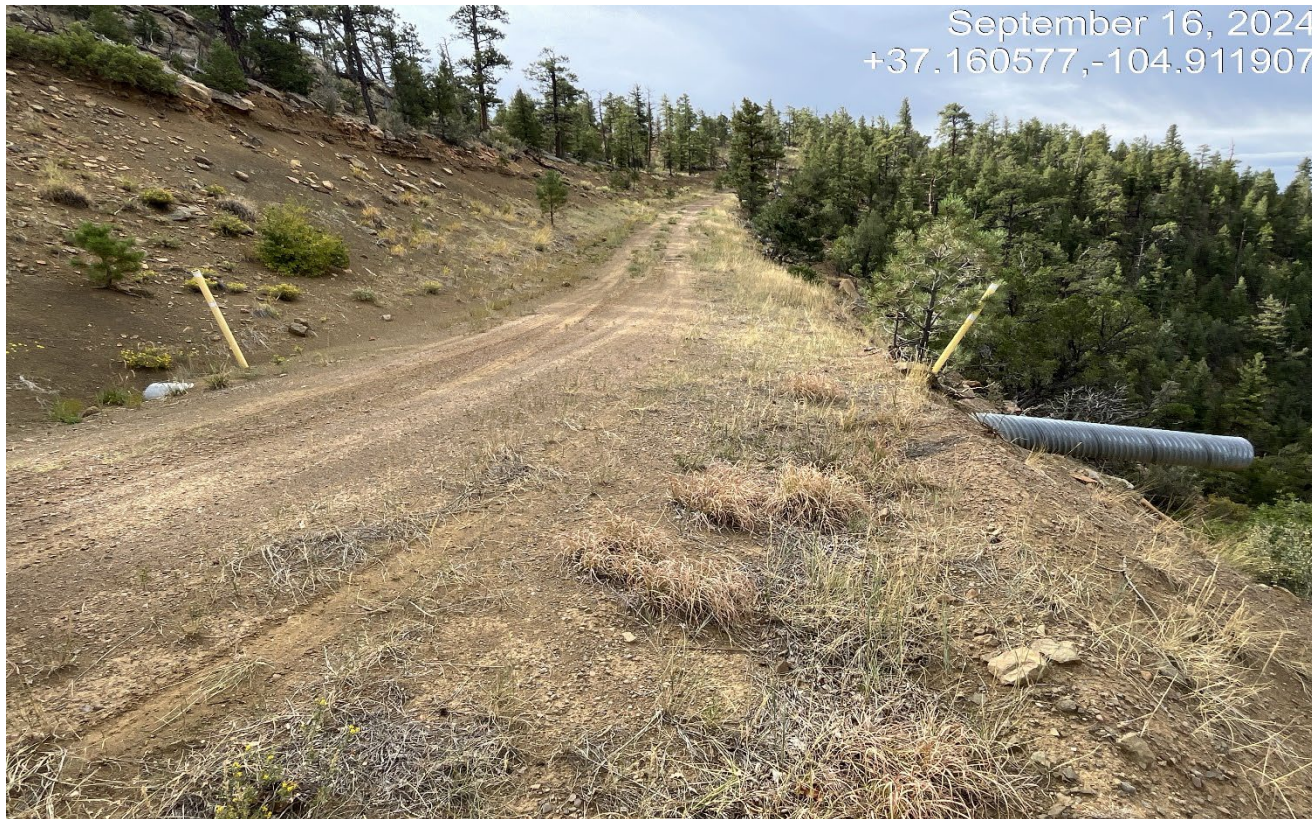
Photo 1. Facing south along the access road to the abandoned wellsite. The culverts will need to be removed and the road recontoured.
