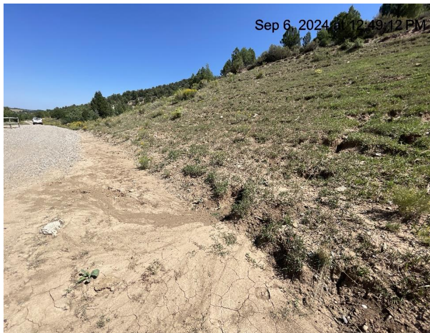
Photo # 8726 Erosion on slope & transport of sediment onto location/insufficient BMP's (east side of location)
