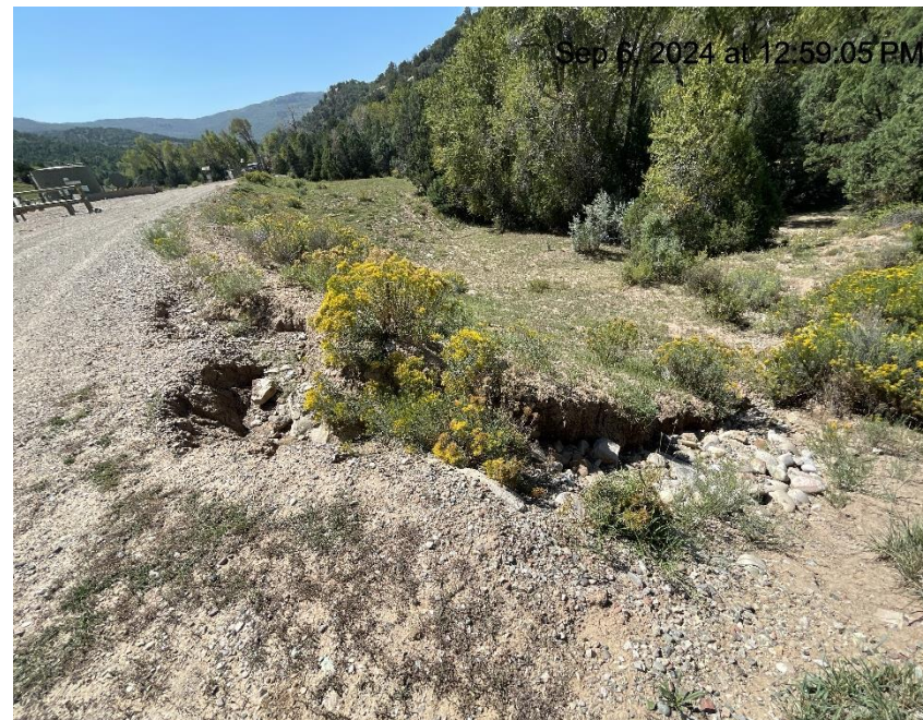
Photo # 8747 Erosion & transport of sediment into a vegetated area/BMP's need maintenance (near entrance to location)
