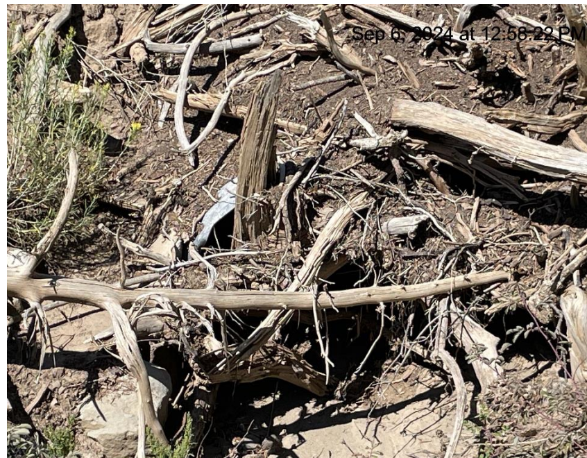
Photo # 8745 Large amount of sediment & debris built up at culvert inlet/capacity of BMP reduced (on lease road near entrance to location
