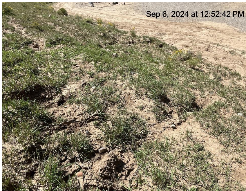
Photo # 8732 Erosion on slope & transport of sediment onto location/insufficient BMP's (east side of location)
