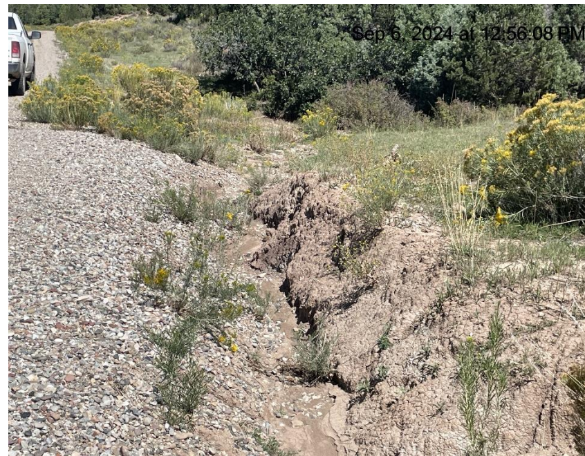
Photo # 8739 Insufficient BMP's/runoff controls in ditch (E/NE area of location near entrance to location)
