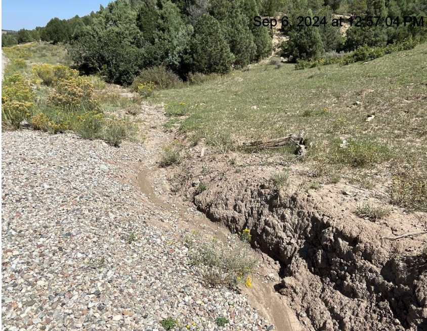
Photo # 8740 Insufficient BMP's/runoff controls in ditch, sediment is being carried off location & into a vegetated area & towards a nearby creek/drainage (NE area of location near entrance to location)
