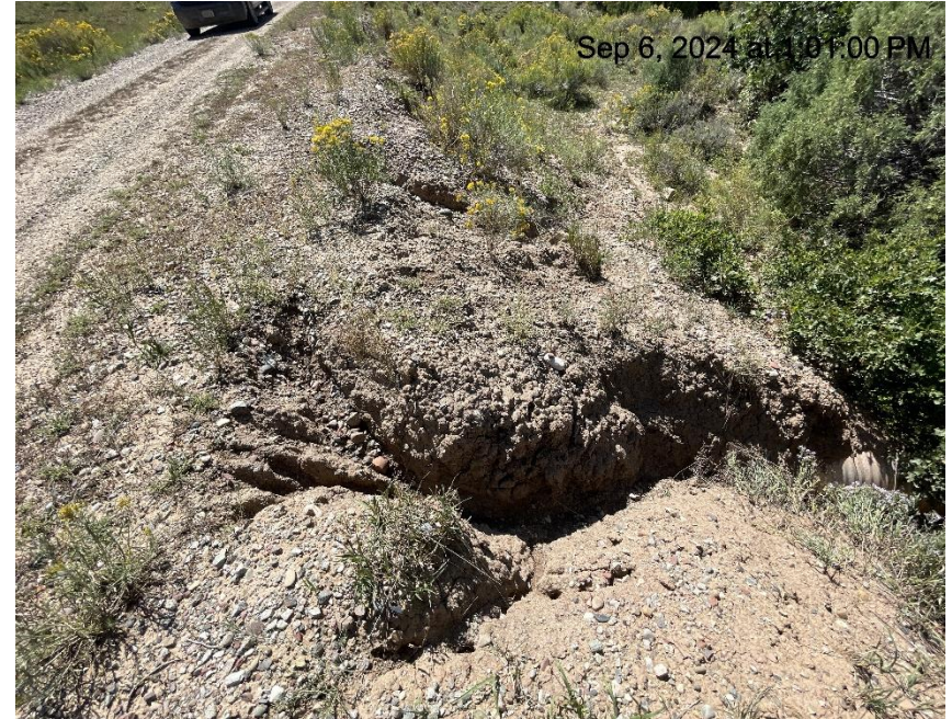
Photo # 8749 Erosion & transport of sediment off edge of lease road (near culvert on lease road near entrance to location)
