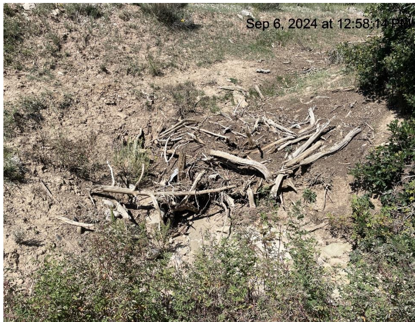
Photo # 8744 Large amount of sediment & debris built up at culvert inlet/capacity of BMP reduced (on lease road near entrance to location
