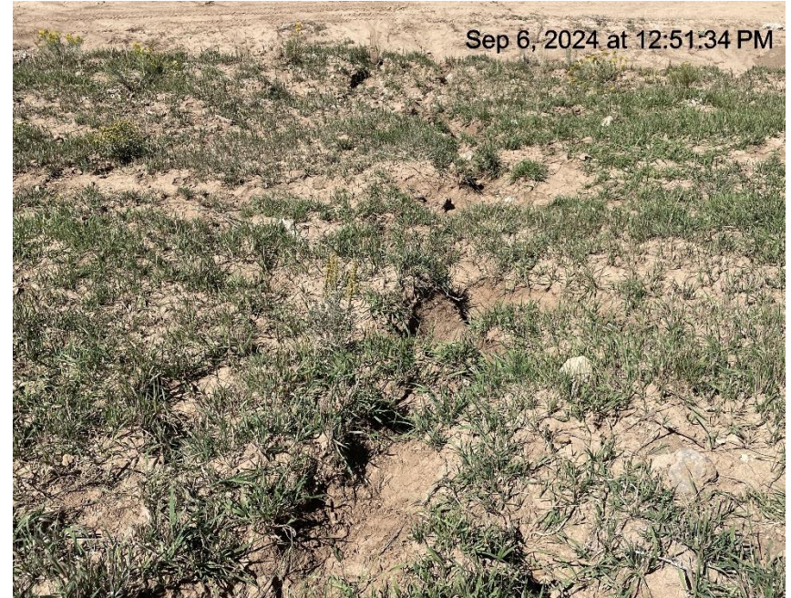
Photo # 8731 Erosion on slope & transport of sediment onto location/insufficient BMP's (east side of location)
