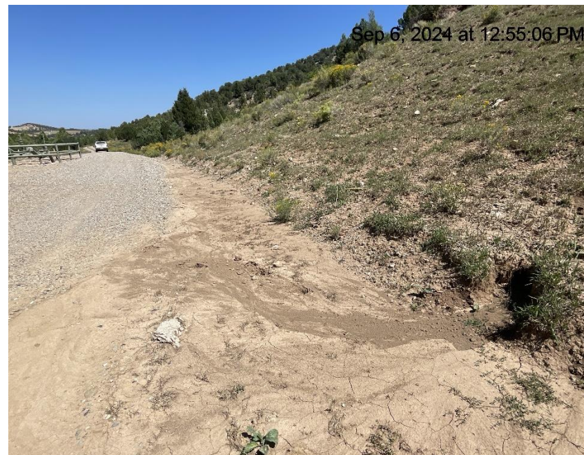
Photo # 8727 Erosion on slope & transport of sediment onto location/insufficient BMP's (east side of location)
