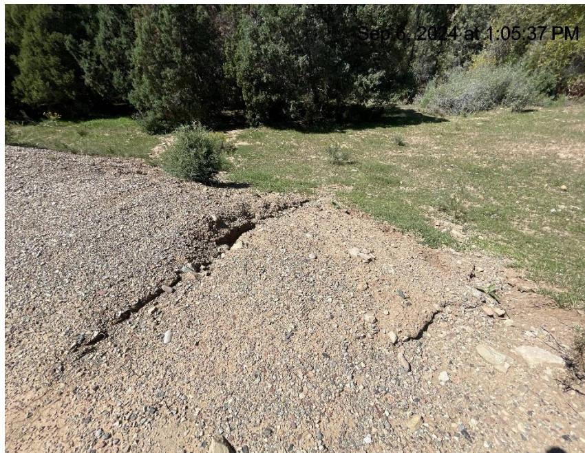
Photo # 8750 Erosion on slope & transport of sediment off location & into a vegetated area (near Summit Midstream meter house)
