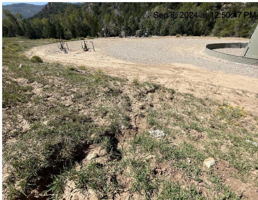
Photo # 8728 Erosion on slope & transport of sediment onto location/insufficient BMP's (east side of location)
