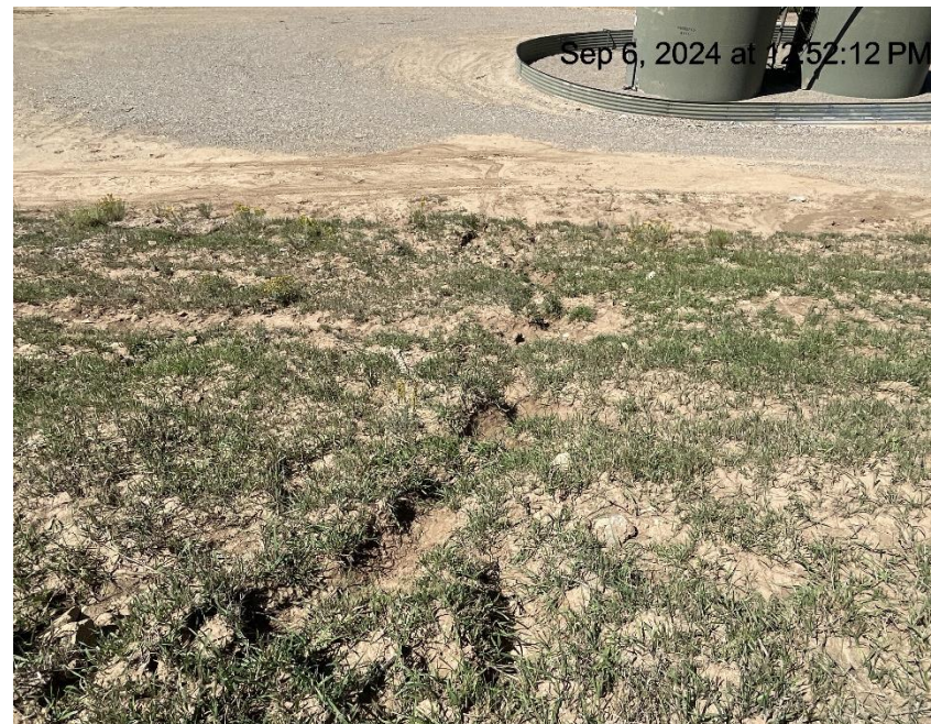
Photo # 8733 Erosion on slope & transport of sediment onto location/insufficient BMP's (east side of location)
