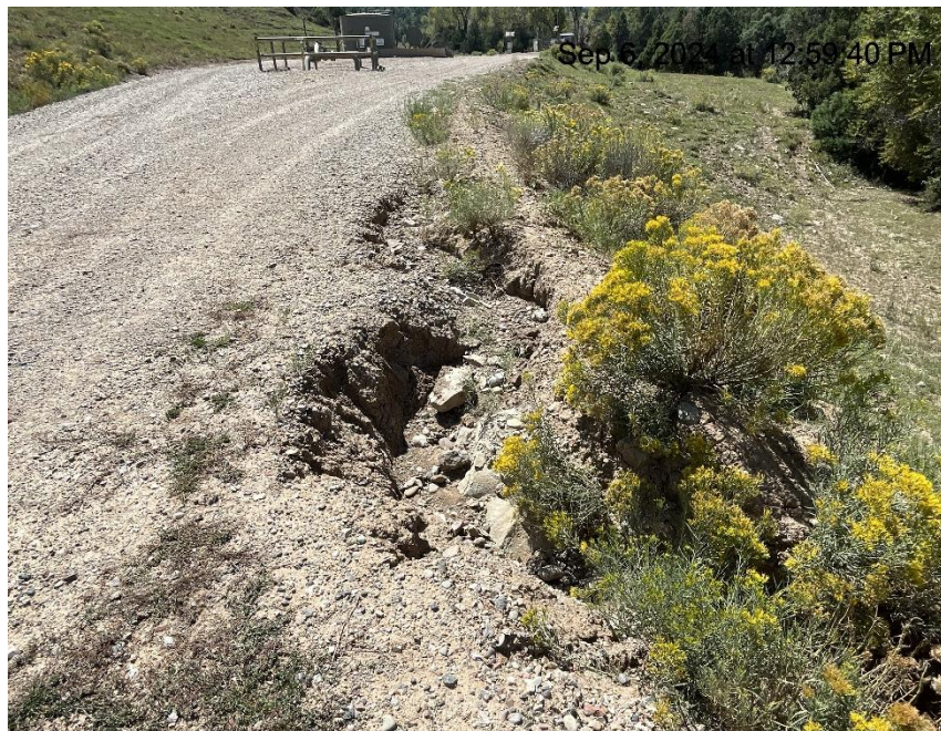
Photo # 8746 Erosion & transport of sediment (near entrance to location)
