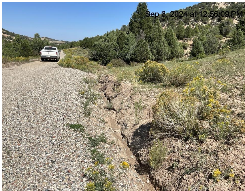
Photo # 8738 Insufficient BMP's/runoff controls in ditch (E/NE area of location near entrance to location)
