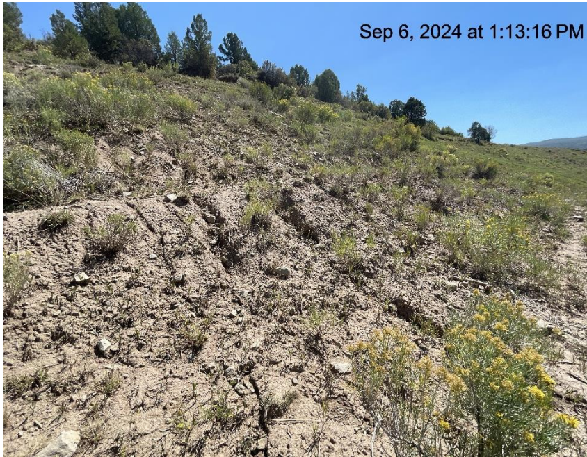
Photo # 8734 Erosion on slope & transport of sediment /insufficient BMP's (E/NE area of location)
