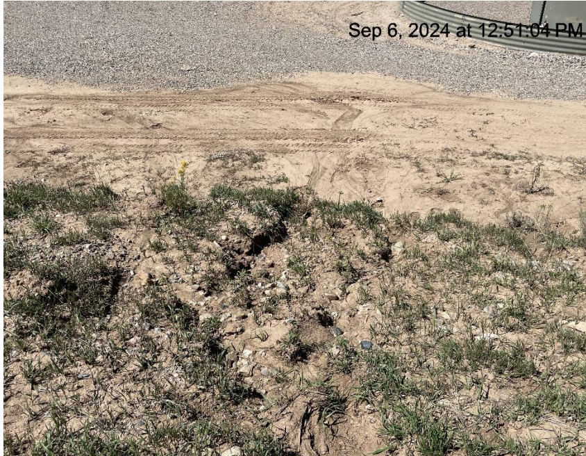
Photo # 8730 Erosion on slope & transport of sediment onto location/insufficient BMP's (east side of location)
