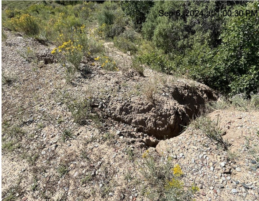
Photo # 8748 Erosion & transport of sediment off edge of lease road (near culvert on lease road near entrance to location)
