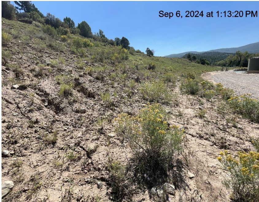
Photo # 8736 Erosion on slope & transport of sediment /insufficient BMP's (E/NE area of location)
