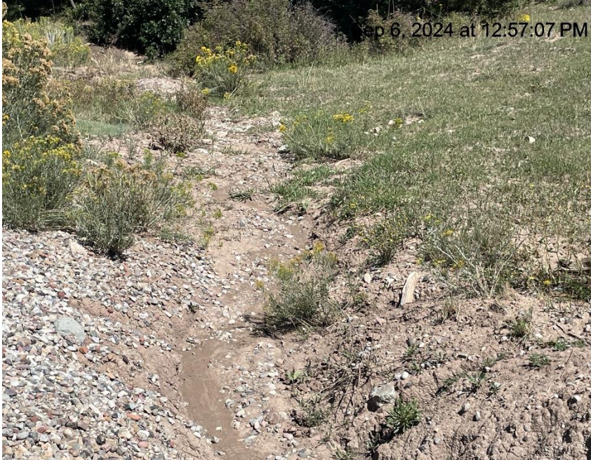
Photo # 8742 Insufficient BMP's/runoff controls in ditch, sediment is being carried off location & into a vegetated area & towards a nearby creek/drainage (NE area of location near entrance to location)
