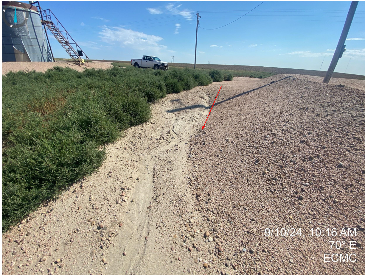
Photo 9. Continued from Photo 8, photo illustrates rill erosion.
