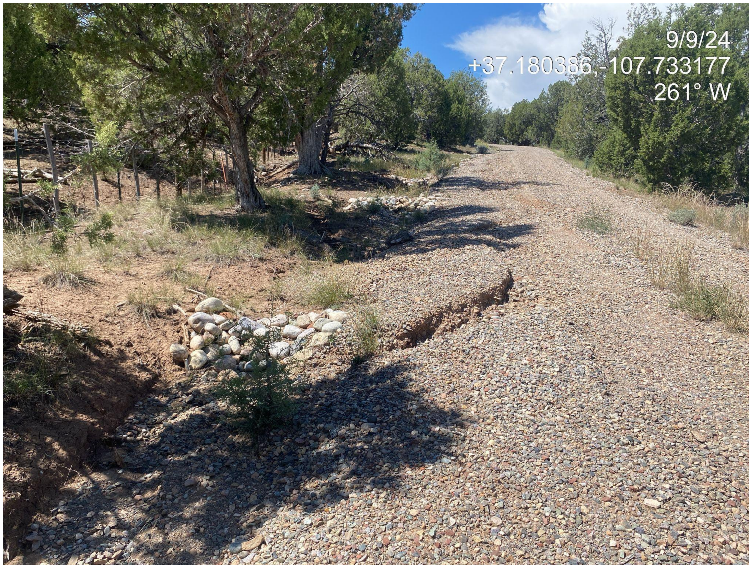
Photo 4. View of erosion forming along the access road. Additional stabilization/Stormwater controls area needed to minimize degradation along the access road.
