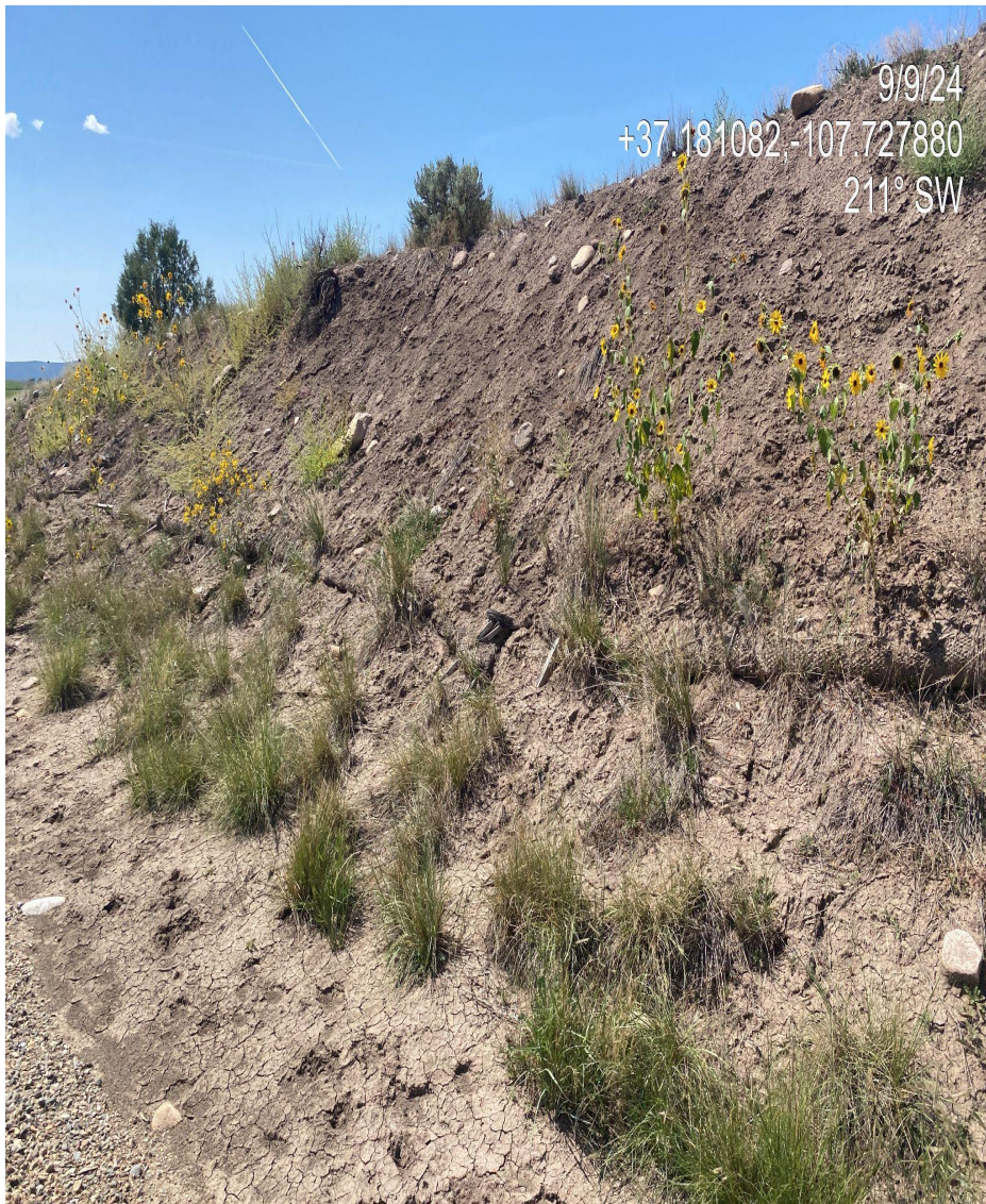
Photo 2. View of storm water controls in the western and northern portions of the cut slope that need maintenance.
