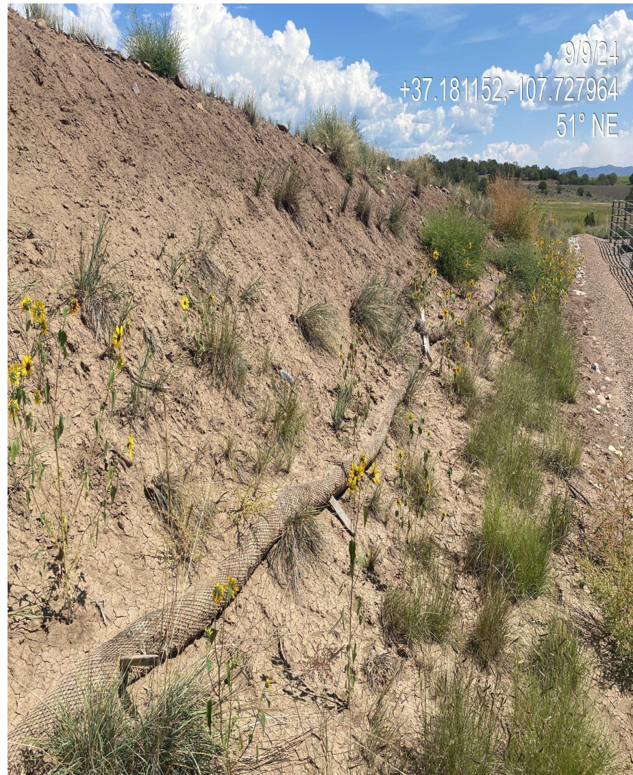
Photo 2. View of storm water controls in the western and northern portions of the cut slope that need maintenance.
