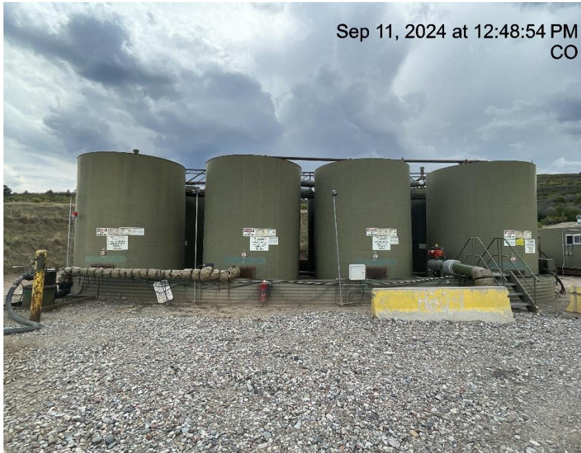
Photo # 9642 Tank battery lacks required signage
