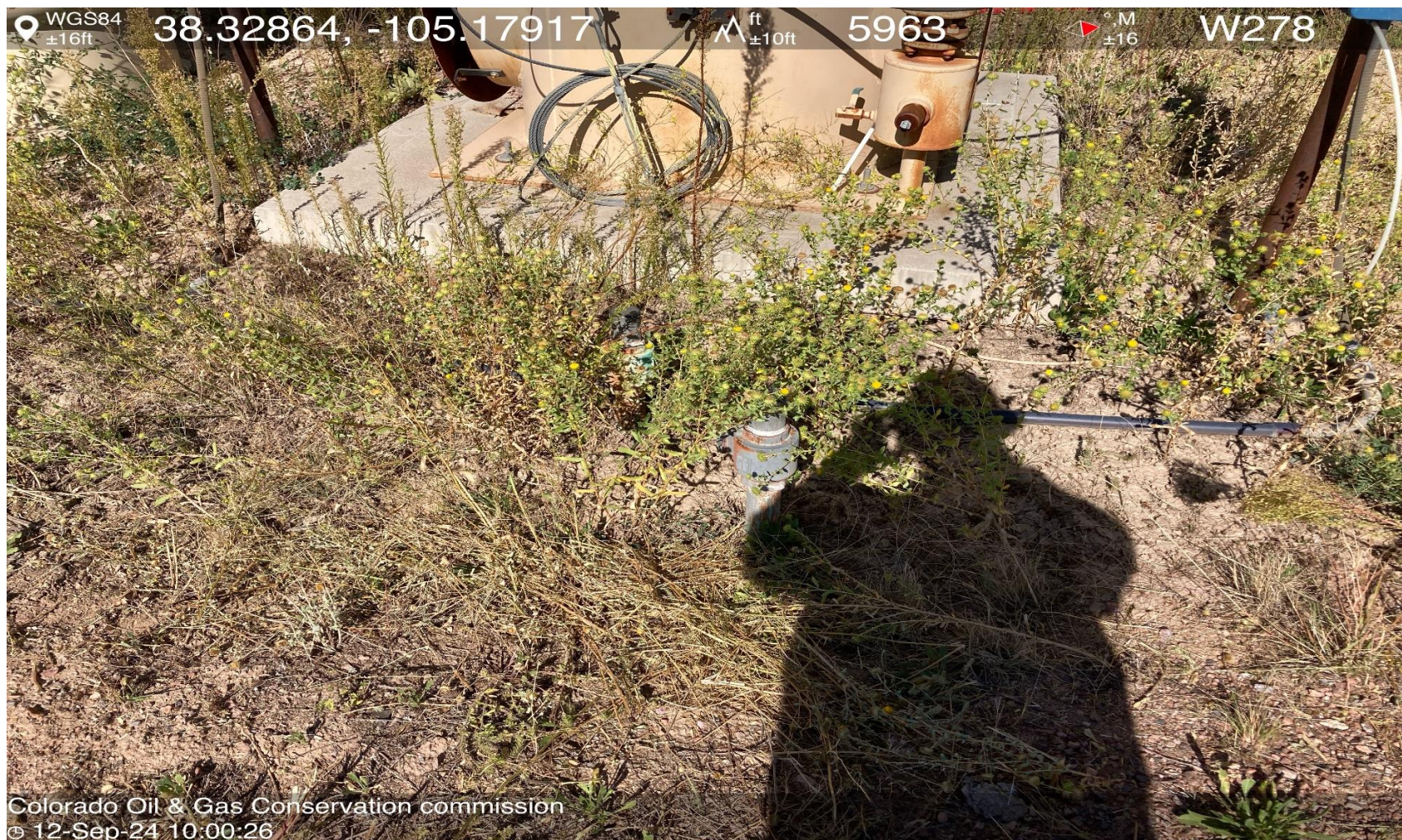
PHOTO 22: UNUSED EQUIPMENT ( UNUSED RISERS BY ECD'S). REMOVE OR MARK UNUSED RISERS PER RULE 606. CA DATE 10-12-2024.
