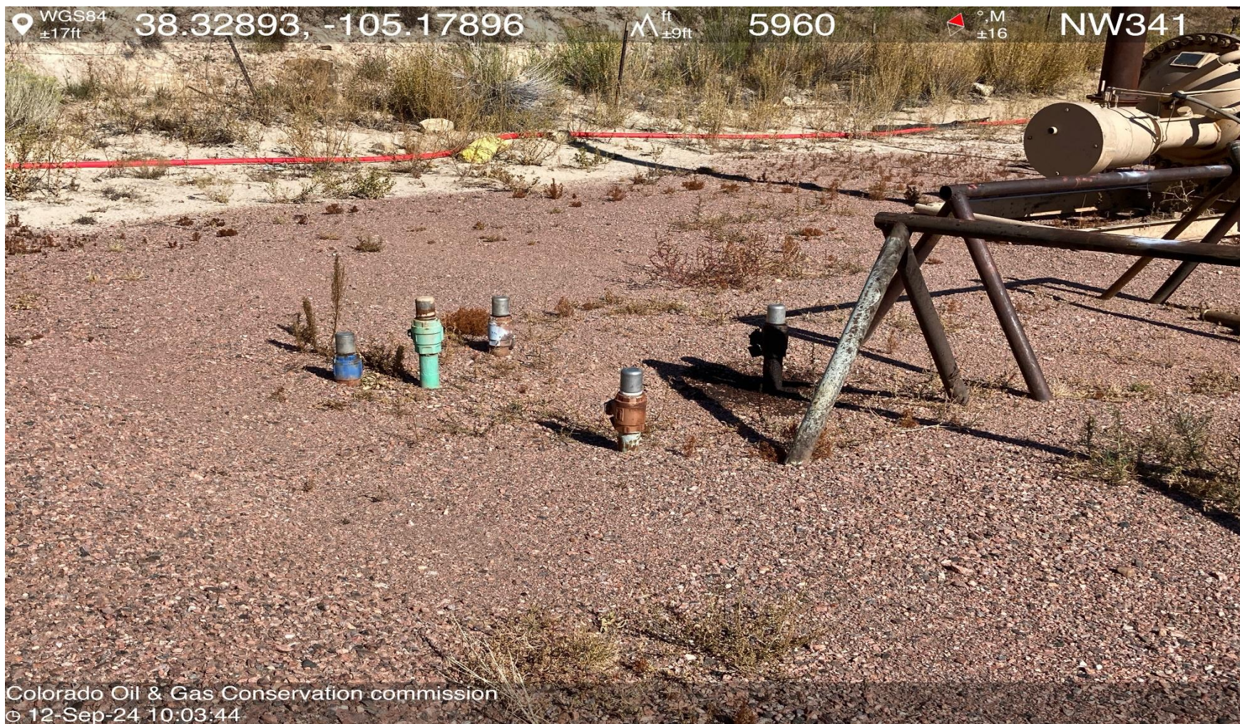
PHOTO 24: UNUSED EQUIPMENT ( UNUSED RISER NEAR HEATED SEPARATOR). REMOVE OR MARK UNUSED RISERS PER RULE 606. CA DATE 10-12-2024.
