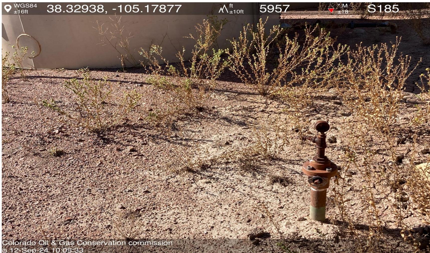
PHOTO 24: UNUSED EQUIPMENT ( UNUSED RISER NEAR CRUDE OIL TANKS). REMOVE OR MARK UNUSED RISERS PER RULE 606. CA DATE 10-12-2024.
