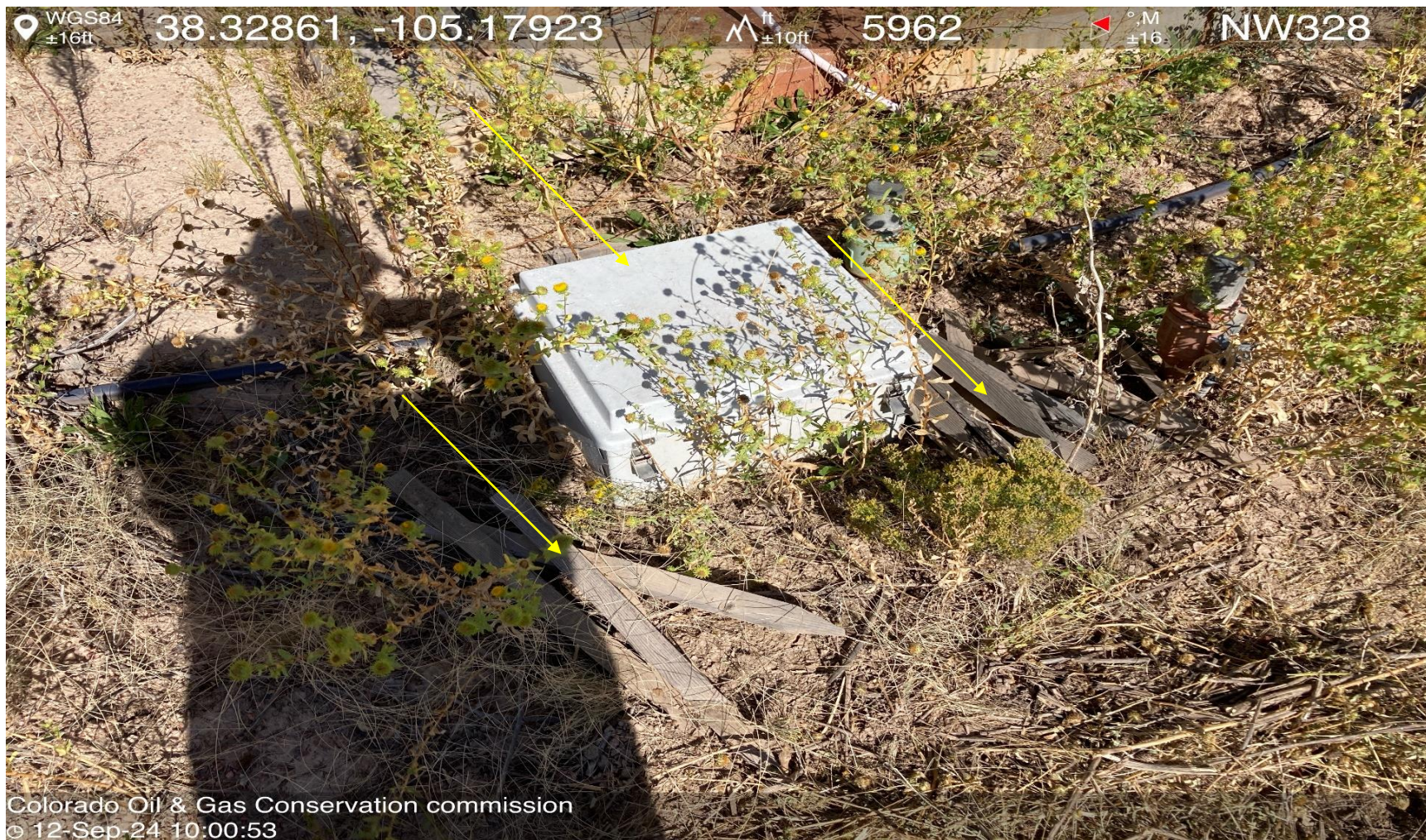
PHOTO 12: UNUSED EQUIPMENT STORED ON LOCATION (EMPTY FIBERGLASS BOX AND SOME WATTLE STAKES). REMOVE ALL UNUSED EQUIPEMENT FROM LOCATION PER RULE 606. CA DATE 9-18-2024.
