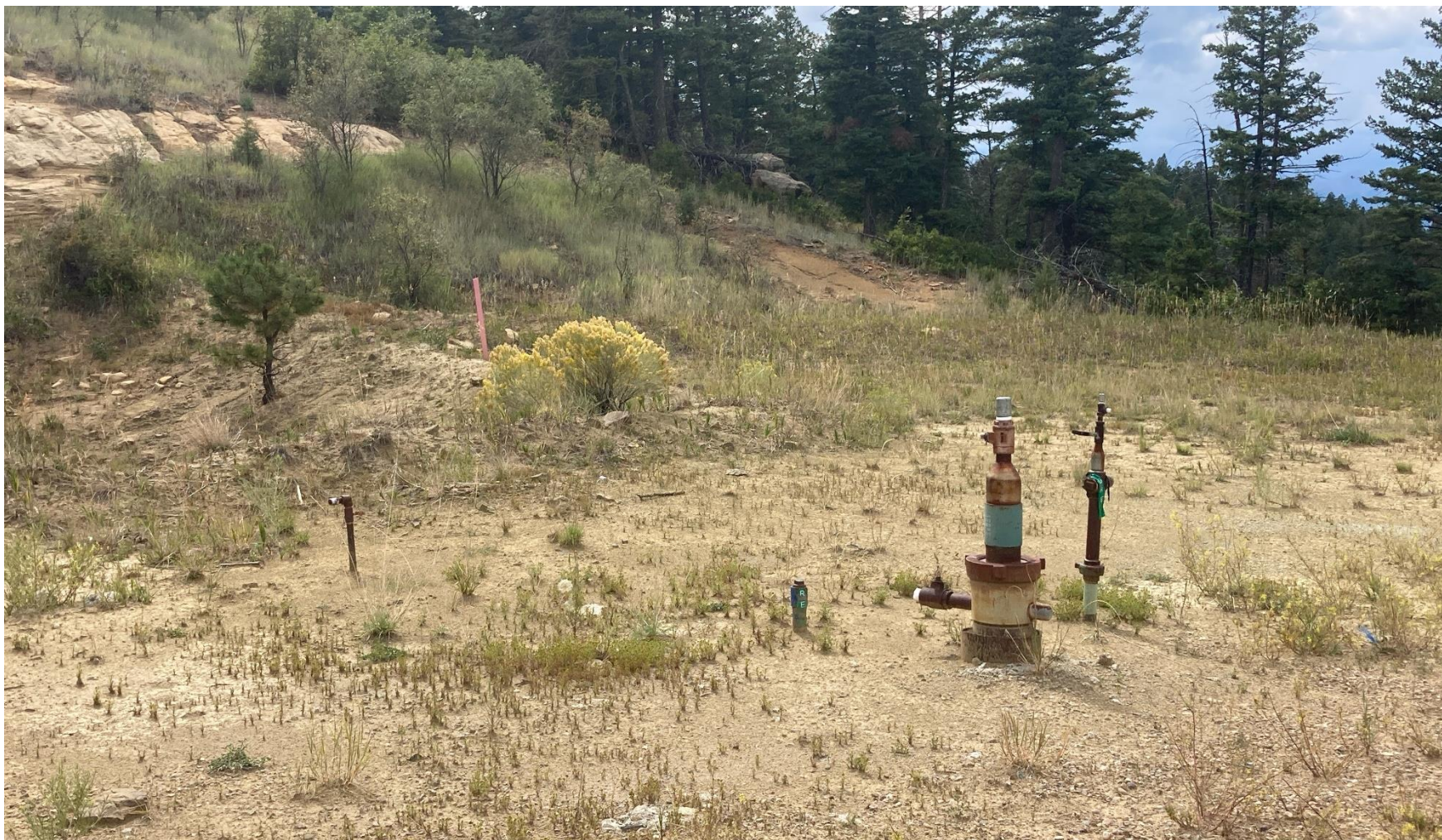
PHOTO 3: UNUSED EQUIPMENT (UNUSED UNMARKED RISERS 1-1" AND 2-2"). REMOVE OR MARK RISERS PER RULE 606. CA DATE 10-12-2024.
