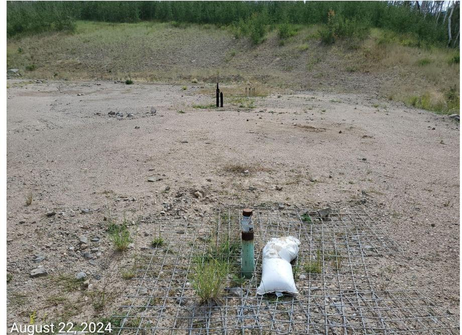
**Photo 1:** Photos examples showing unused riser equipment remains on the Location. Risers require removal.
