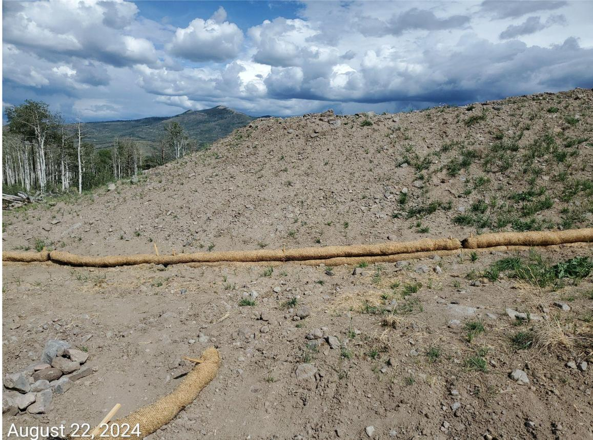
**Photo 5:** Photo taken from the fill slopes. Slopes on the north end of the Location remain predominantly bare; Operator has since stacked a 2nd erosion log on top of the wattles previously placed, however, BMPs to minimize erosion and degradation at the slope not been implemented.
