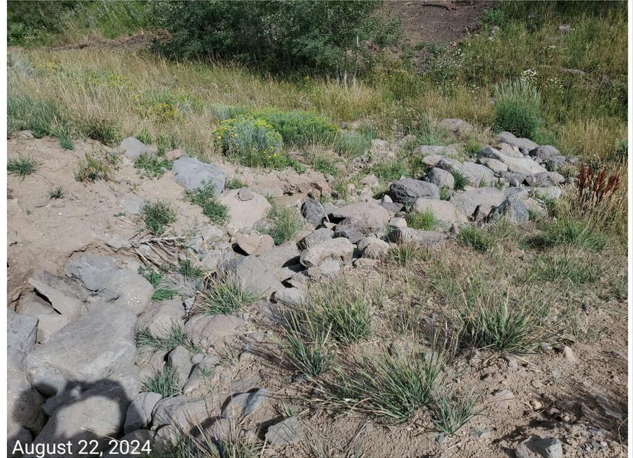
**Photo 3:** Photos taken from the east end of the Location. Outlets on the north and east end of the Location have not been installed or maintained per good engineering practice; geotextile lining in conjunction with multiangular rip-rap material has not been implemented per good engineering practice; stormwater degradation to the walls of the outlets has persisted.
