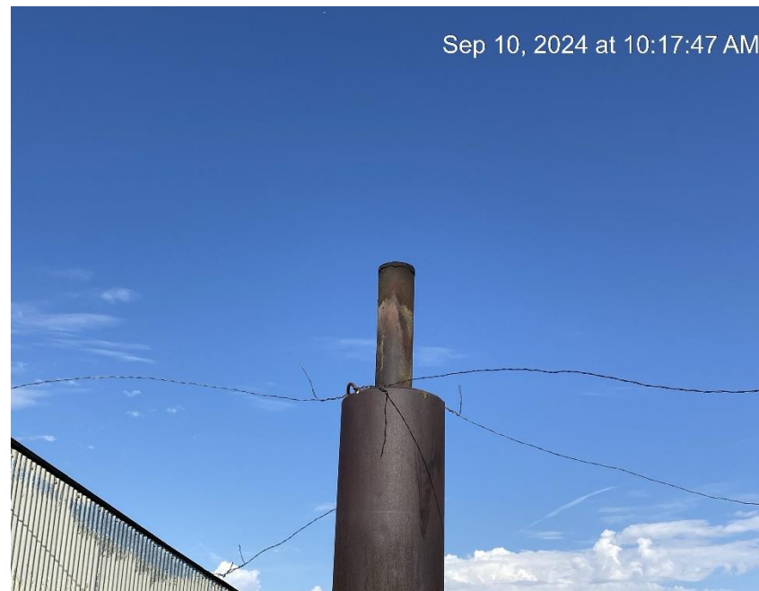
Stack missing bird protection
