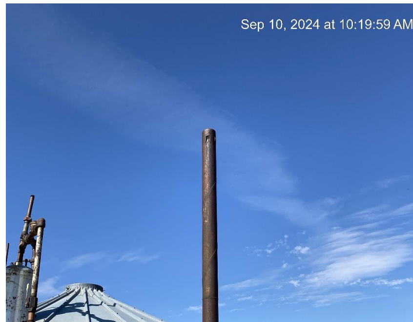
Stack missing bird protection
