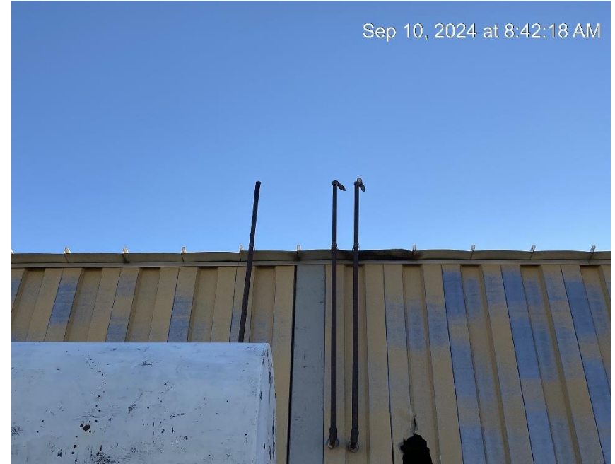
Riser missing protective cap
