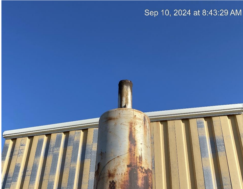
Stack lacking bird protection
