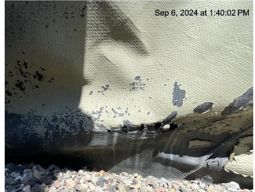
Photo # 9017 Multiple holes in liner/liner needs maintenance
