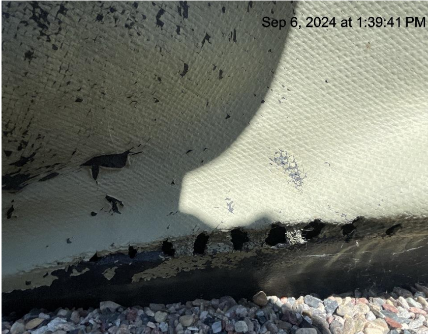
Photo # 9016 Multiple holes in liner/liner needs maintenance
