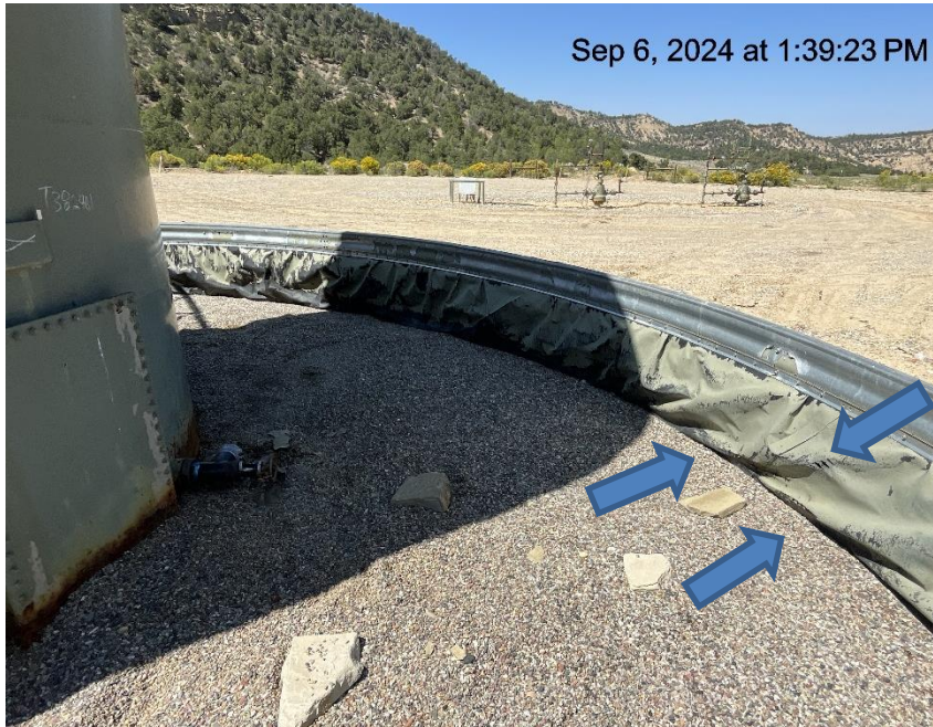
Photo # 9014 Multiple holes in liner/liner needs maintenance
