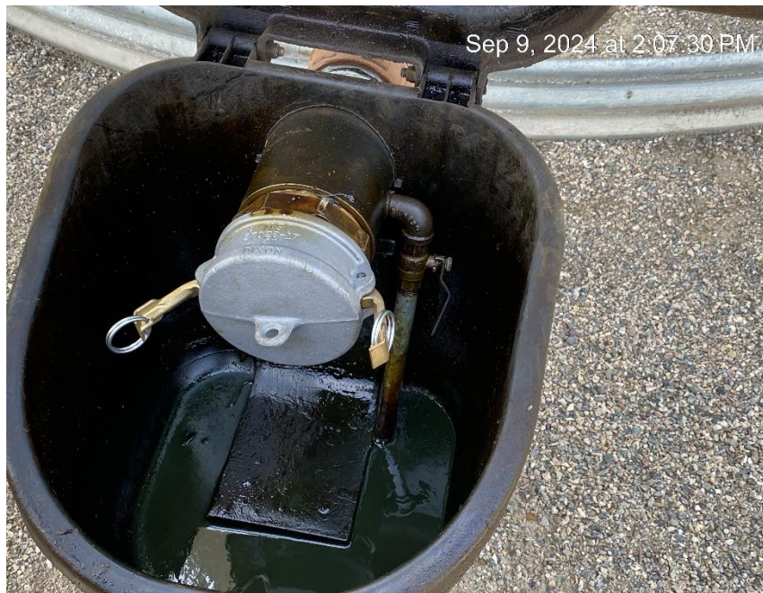
Side valve open. Load line was double-valved.
