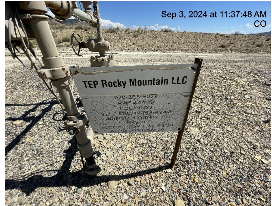
Photo # 7652 RWF 444-19 wellhead sign cracking & peeling
