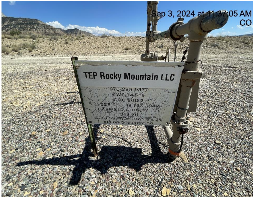
Photo # 7651 RWF 344-19 wellhead sign cracking & peeling
