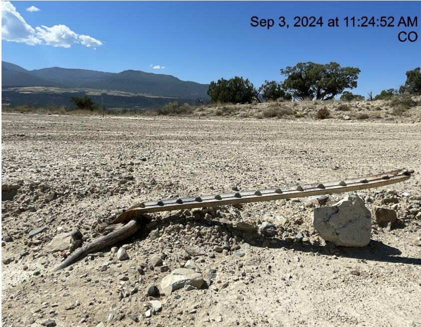
Photo # 7655 Improperly marked deadman
