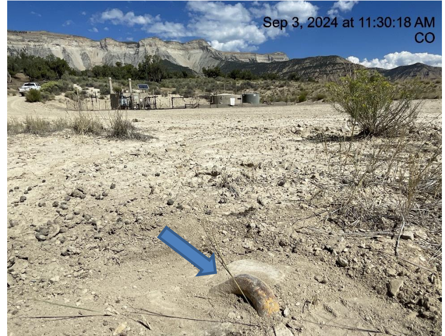
Photo # 7658 Same unmarked deadman from a different angle
