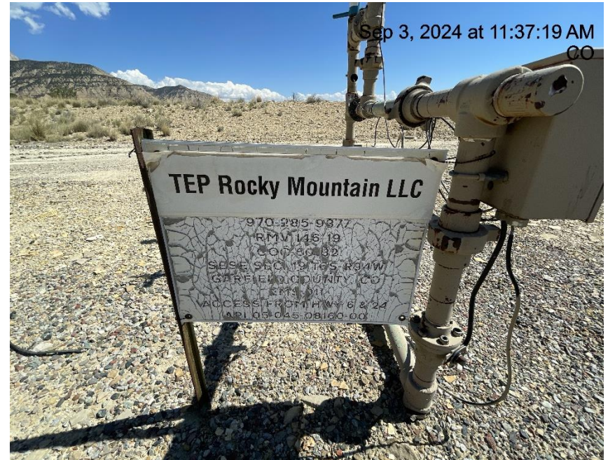
Photo # 7650 RMV 146-19 wellhead sign cracking & peeling/some required info starting to become illegible
