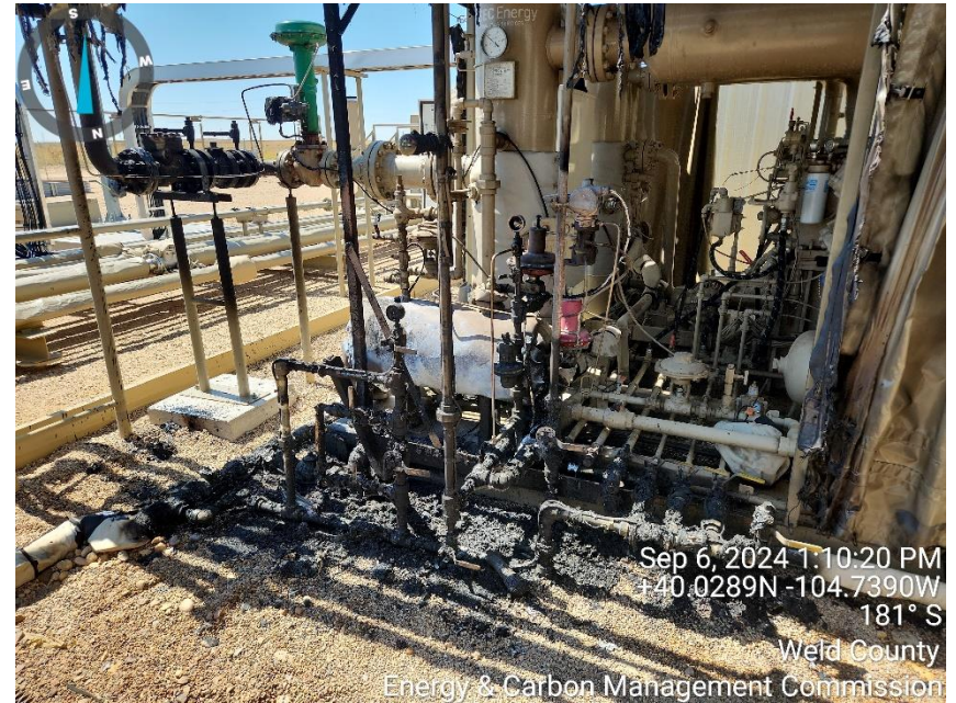
Photo 2 fire area on compressor skid
