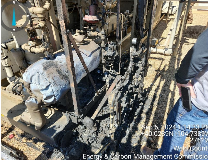
Photo 1 fire area on compressor skid
