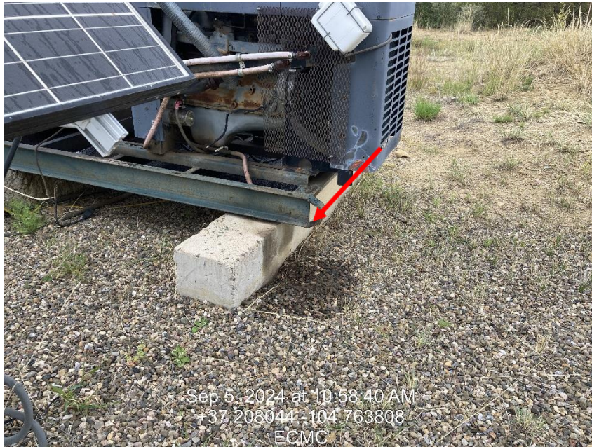
Photo 5 – Oil Stained soils at engine skid
