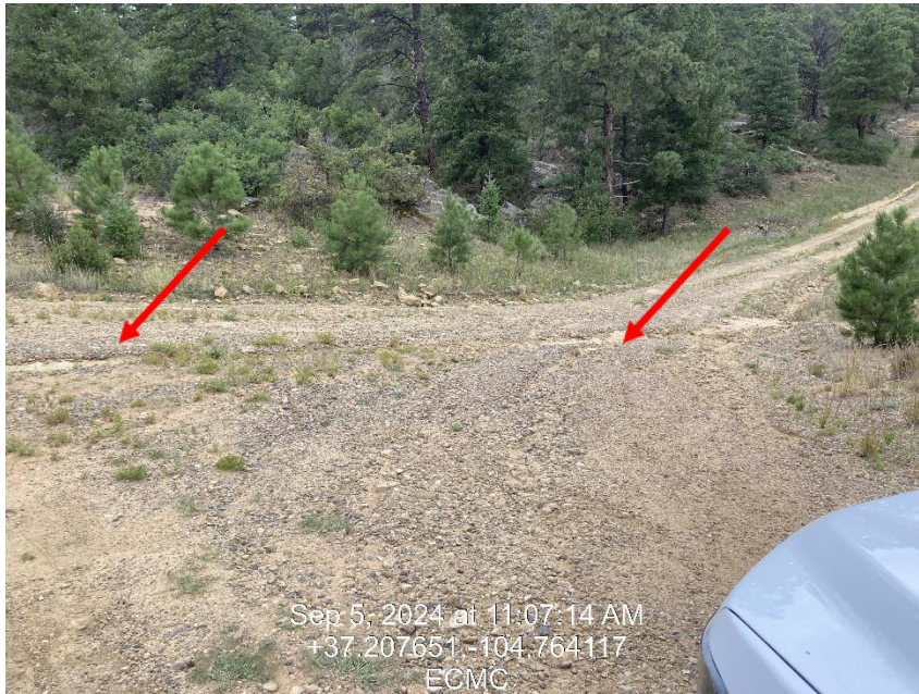
Photo 7 – Stormwater is causing erosion at road intersection
