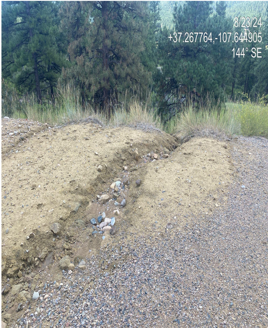
Photo 2. Gully erosion observed forming in the southern interim reclamation area, stabilization/control measures needed in this area.
