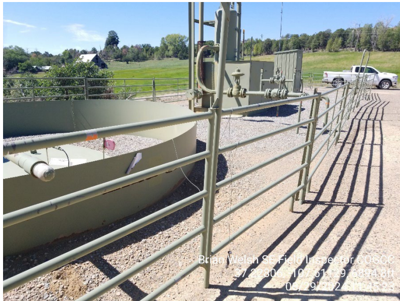
3. Production equipment. Tank label has peeled off
