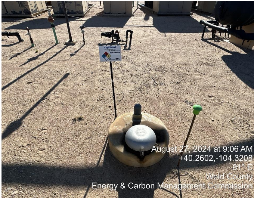
Missing Capacity Label
