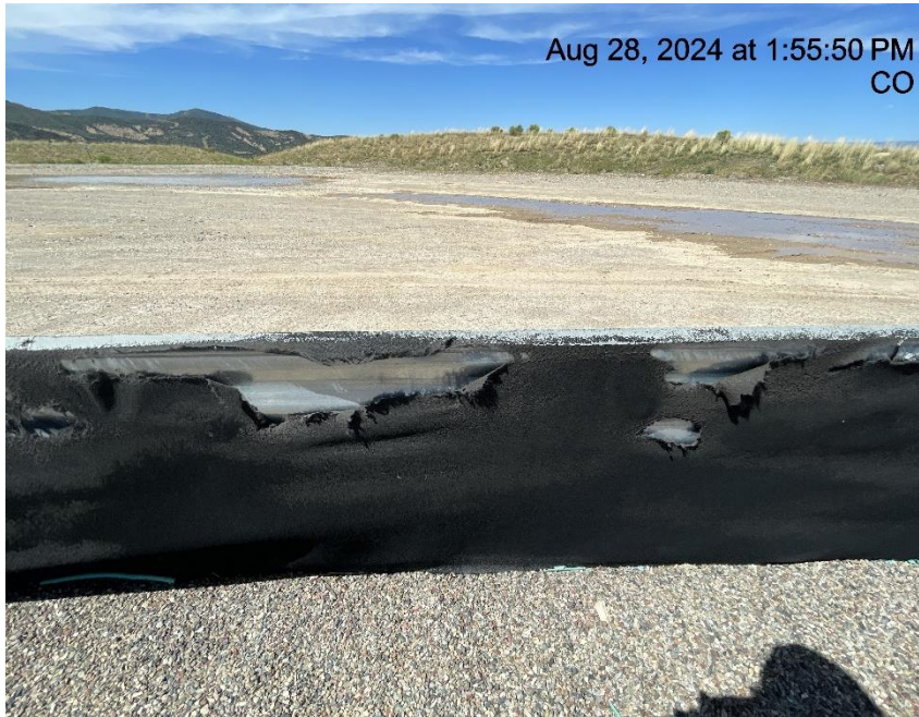
Photo # 7035 Secondary containment liner needs maintenance
