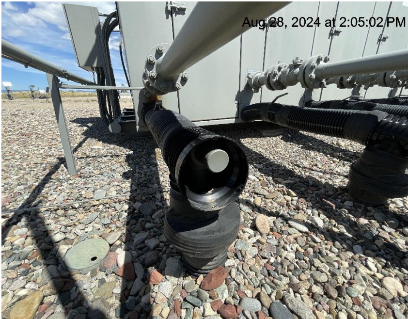
Photo # 7033 Flowline heating insulation open ended/open to entry by wildlife/wildlife hazard
