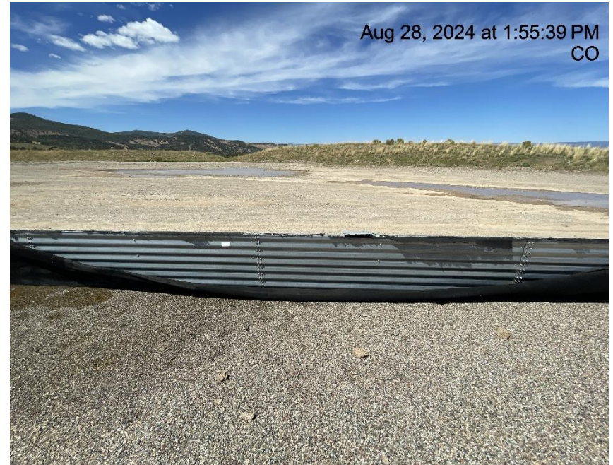
Photo # 7034 Secondary containment liner needs maintenance
