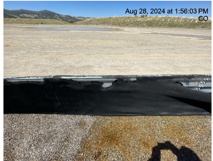
Photo # 7036 Secondary containment liner needs maintenance
