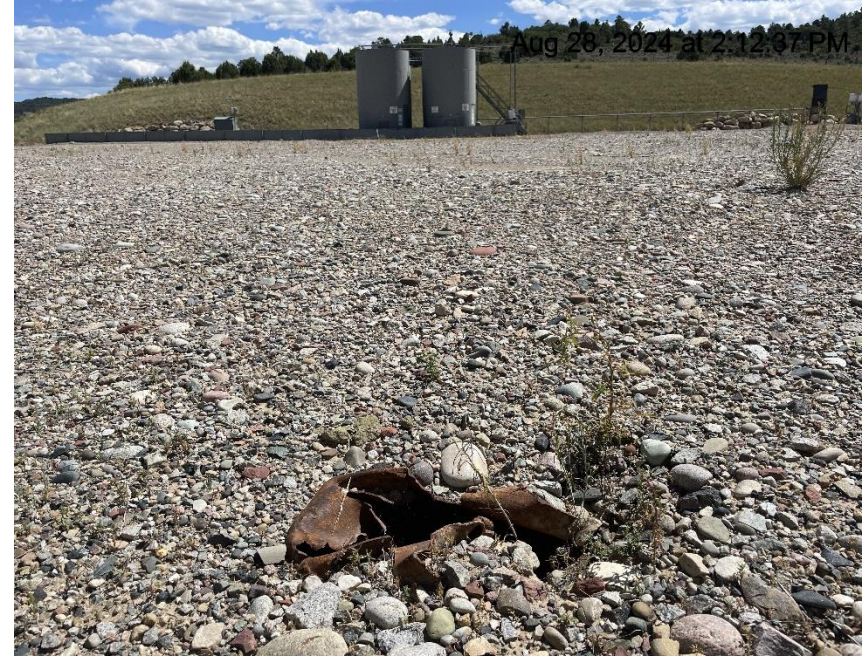
Photo # 7032 Open pipe/wildlife hazard
