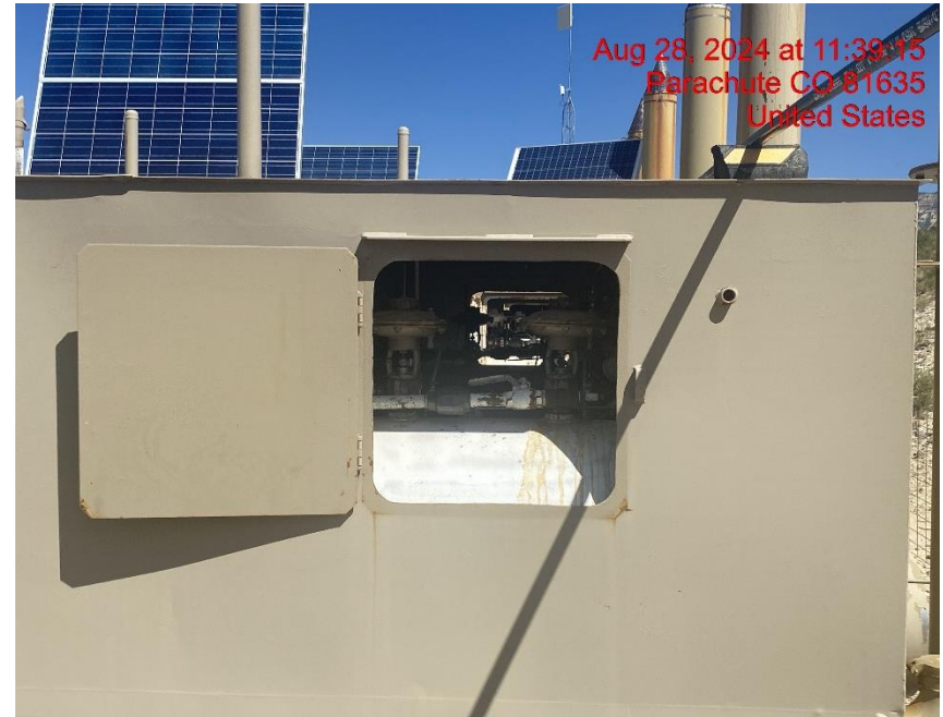
Unsecured Separator/Wildlife Entry Hazard – Photo #03058
