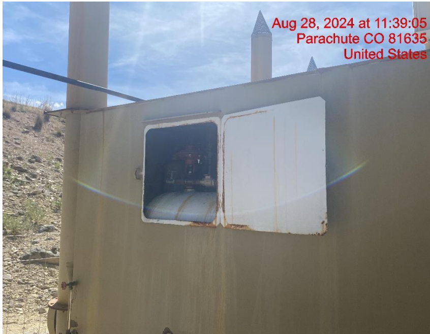
Unsecured Separator/Wildlife Entry Hazard – Photo #03057
