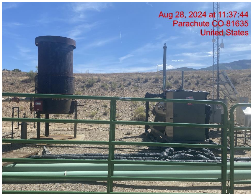
ECD/Heater Treater – Photo #03055
