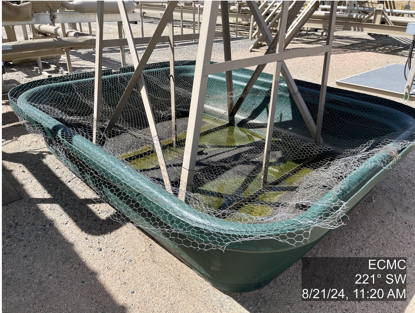
Photo 7. The photo was taken at the well location facing Southwest. The photo illustrates wildlife protections on secondary containment are not secured.
