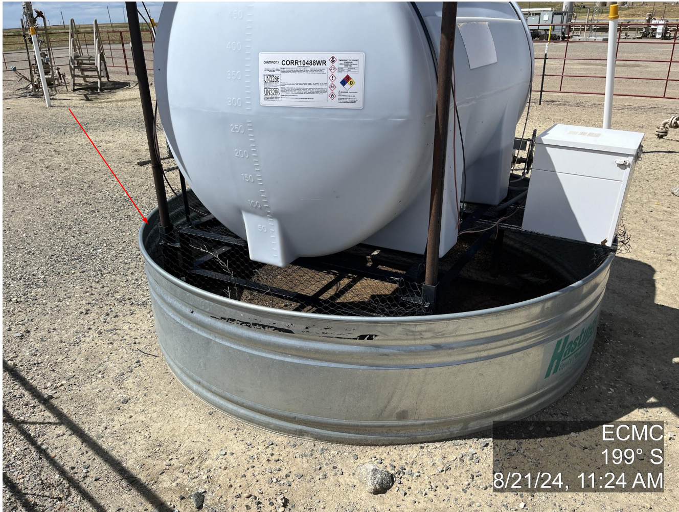
Photo 9. The photo was taken at the well location facing South. The photo illustrates the netting around the secondary containment of a tank has not been installed correctly, not extending over the edge of the tank, and could lead to more wildlife mortality.
