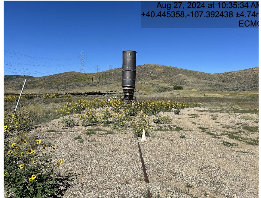
Tank not labeled and not in containment
