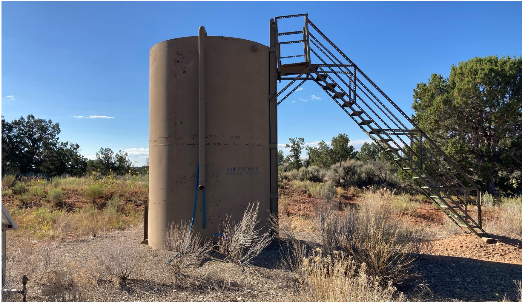
PHOTO 5: NON POTABLE FRESH WATER TANK BATTERY.
