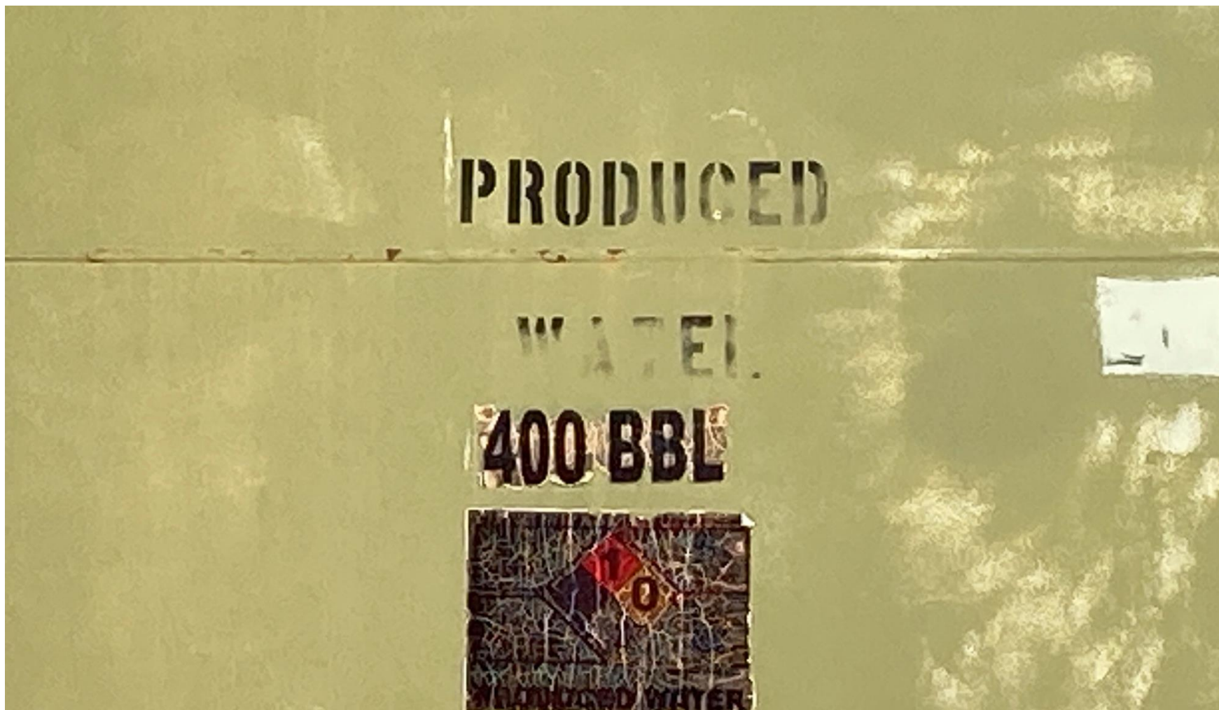
PHOTO 5: NFPA PLACKARD IS BURNT AND IS BARELY LEDGIBLE. POST NFPA PLACARDS PER RULE 605.
