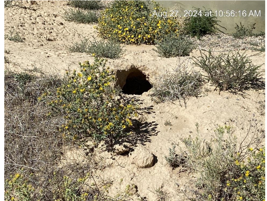
Berm not impervious to spill
