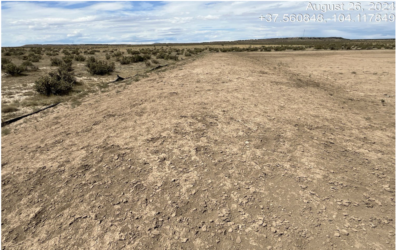
Photo 5. Facing toward the soil stock pile. The topsoil has not been seeded and stabilized and weeds are beginning to establish. There is erosion occurring along the topsoil pile and the silt fence is in disrepair.
