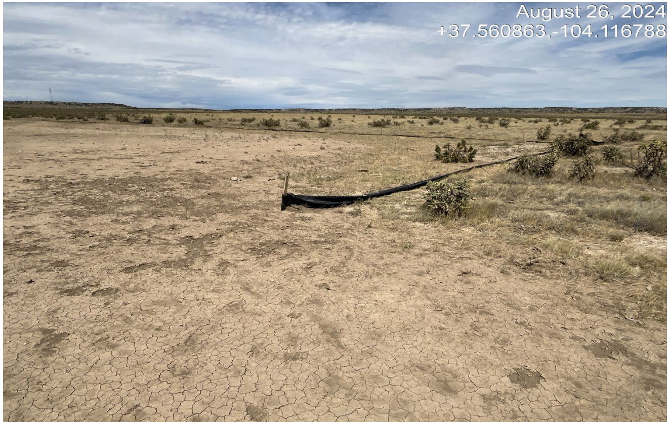
Photo 7. Facing northwest toward the north side of the location. The silt fence is down and not maintained around the entire location.
