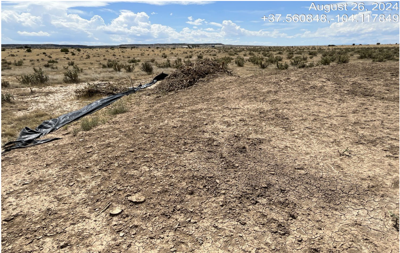
Photo 4. The silt fence is down and not maintained.
