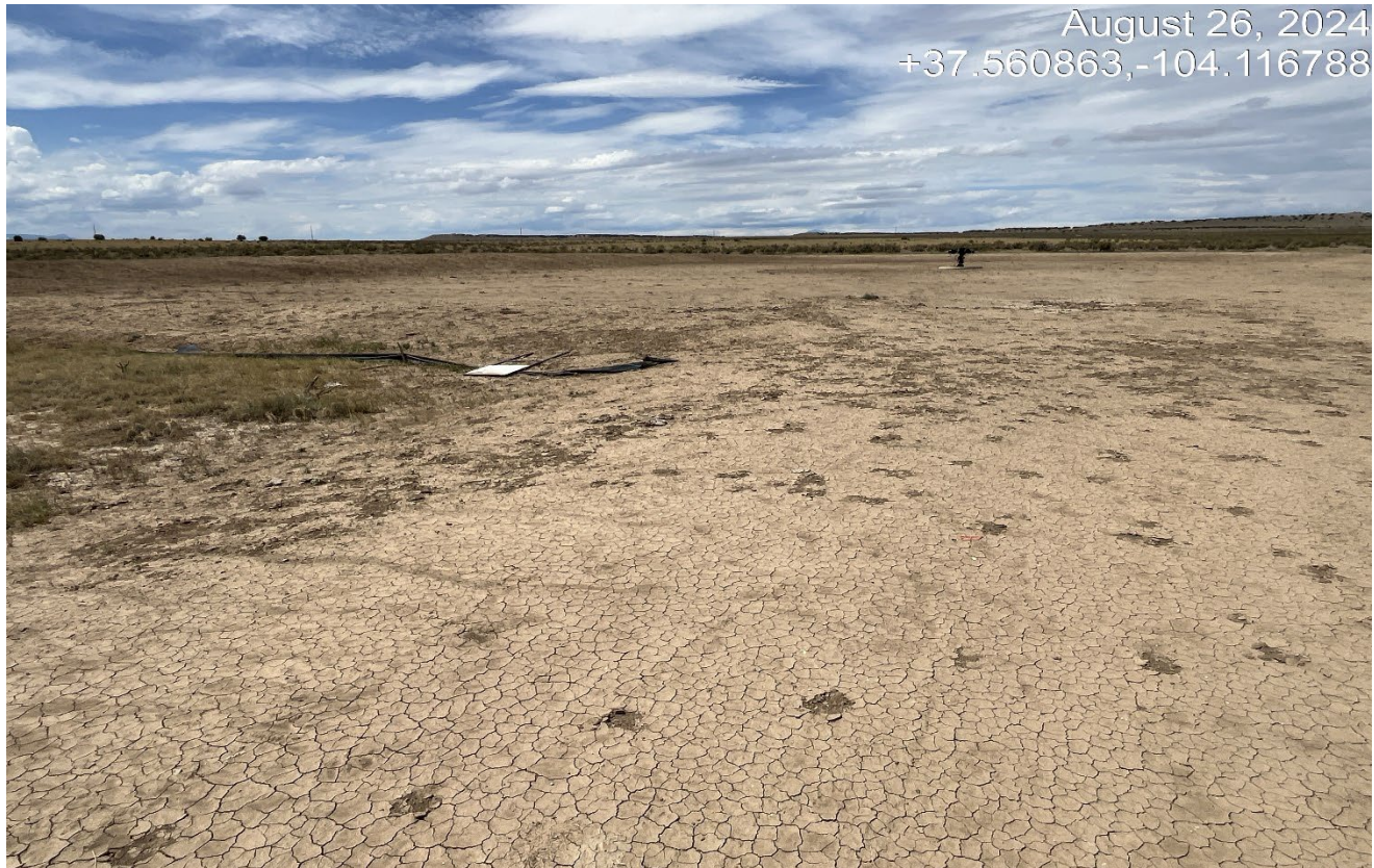
Photo 3. Facing west toward the location. The sign has fallen over and the silt fence is down and not maintained.
