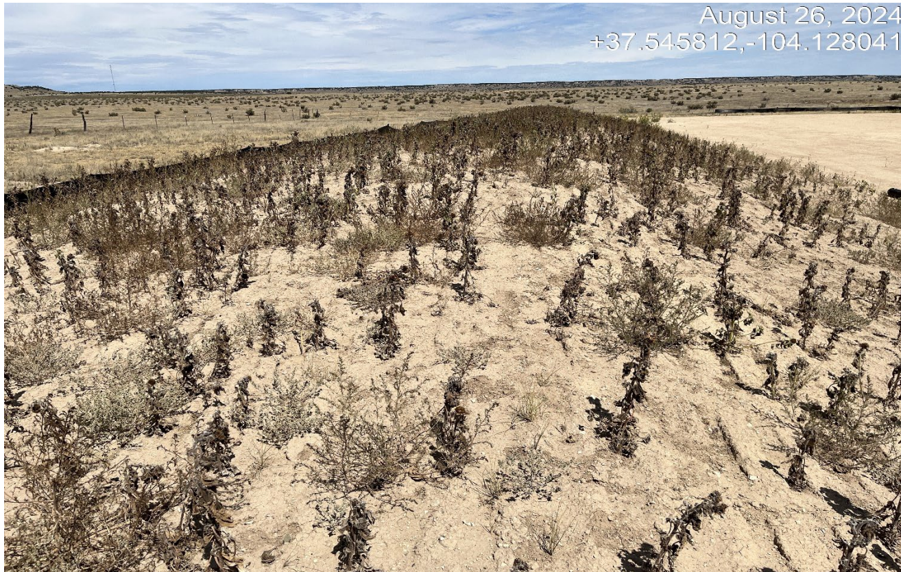
Photo 6. Facing toward the soil stock pile. The topsoil has not been seeded and stabilized and there are weeds established along the topsoil.
