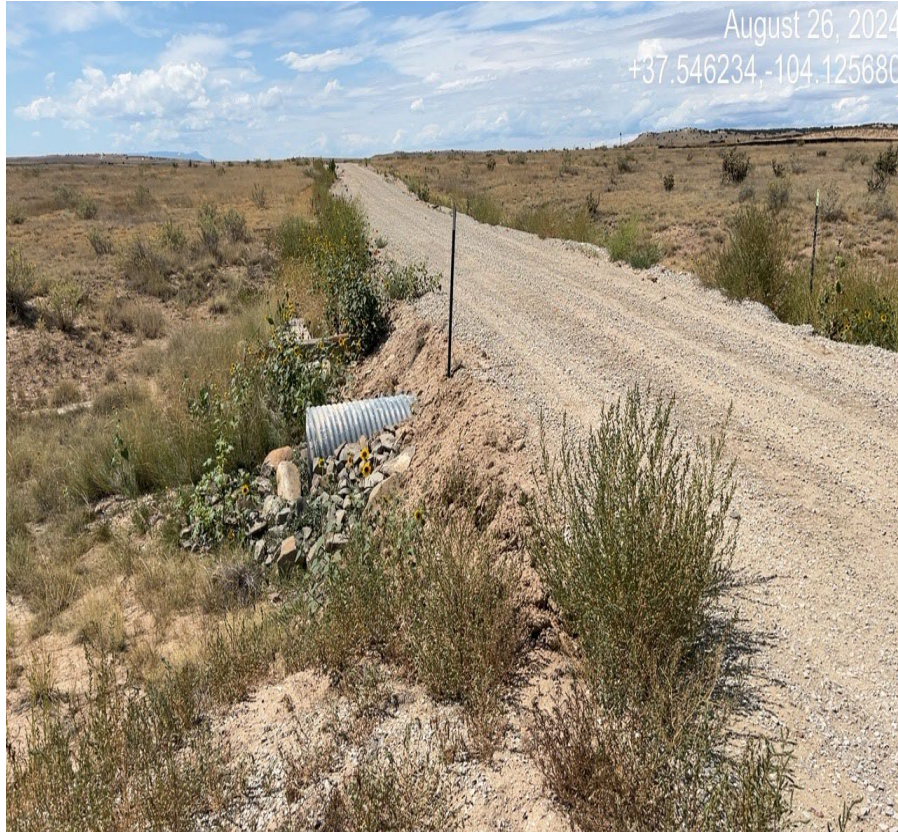
Photo 2. The culvert outlet has been repaired and outlet protection was installed, The loose soil along the embankment need to be stabilized..
