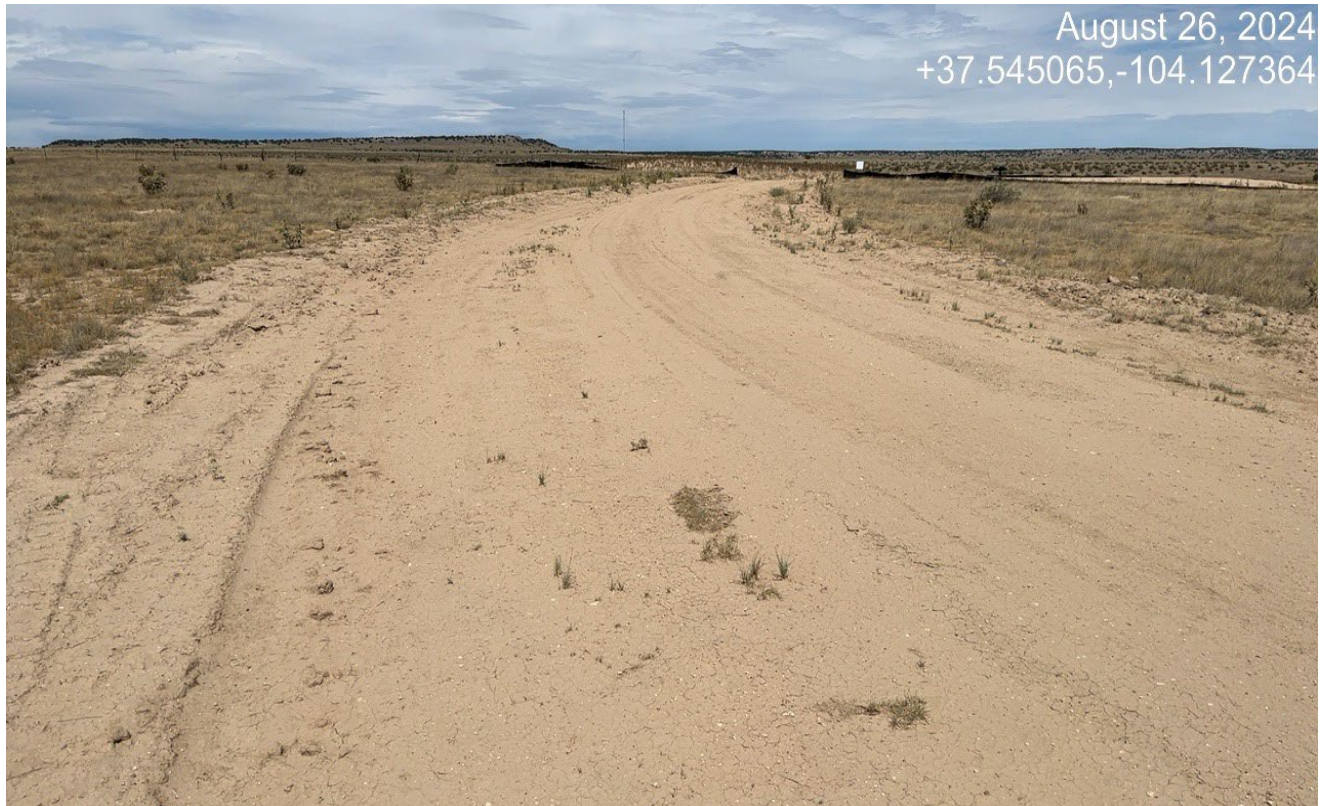
Photo 3. Facing northwest toward the access road. The side of the road needs to be seeded and stabilized. Previous corrective action was not completed.
