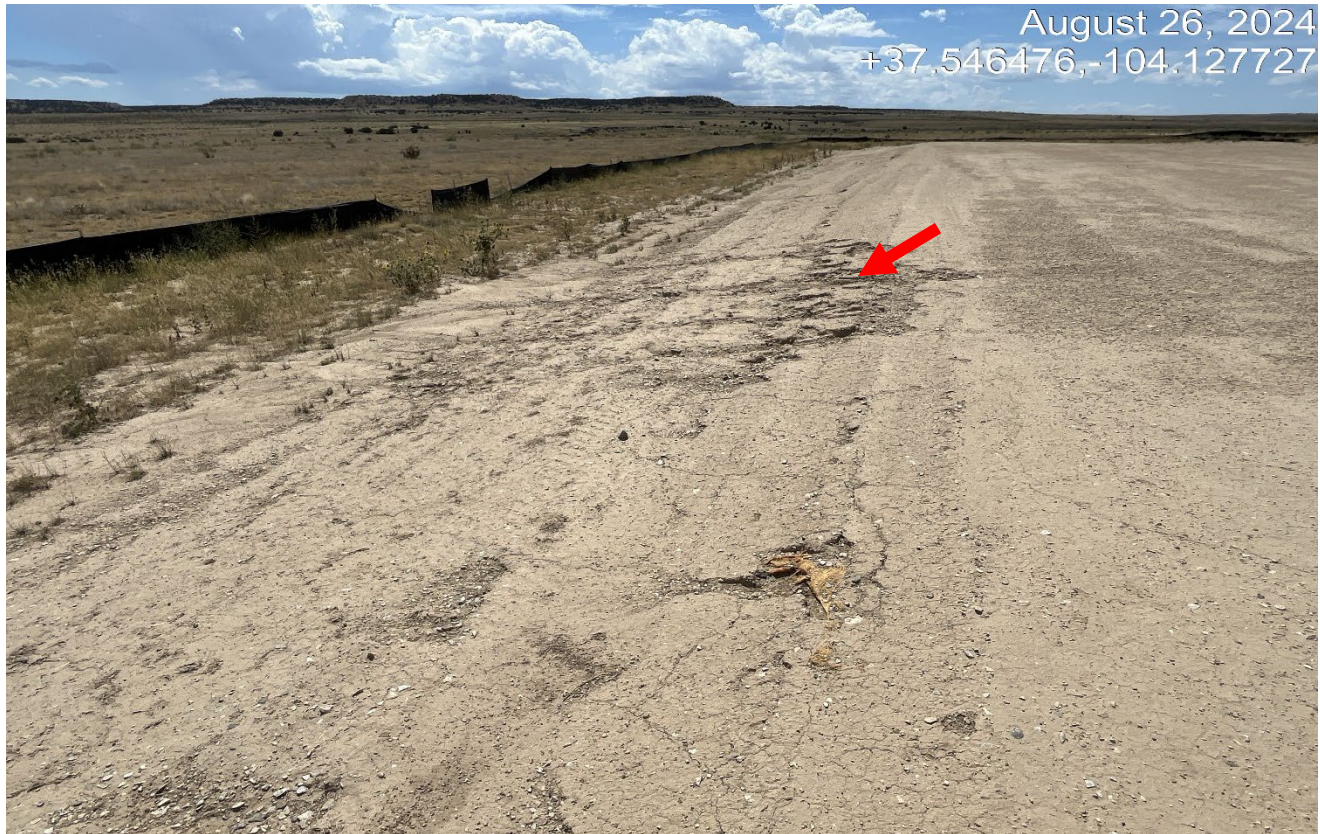
Photo 8. Facing southeast along the fill slope. There is erosion occurring shown at red arrow.
