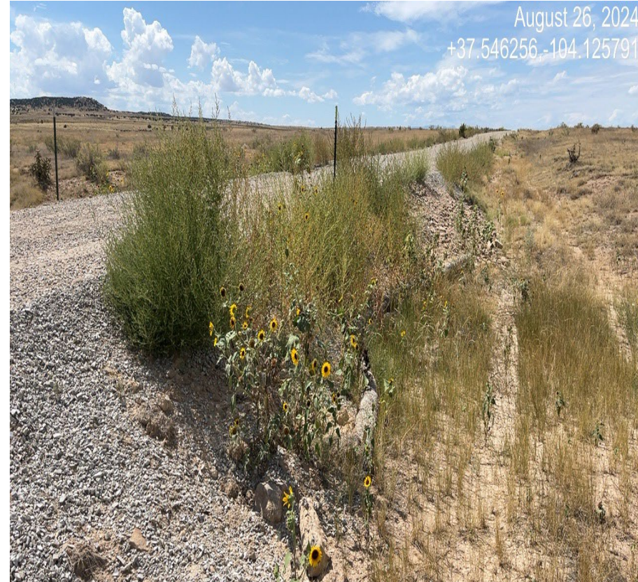
Photo 3. The embankment along the road side at the culvert is not stabilized and loose gravel is falling into the culvert.
