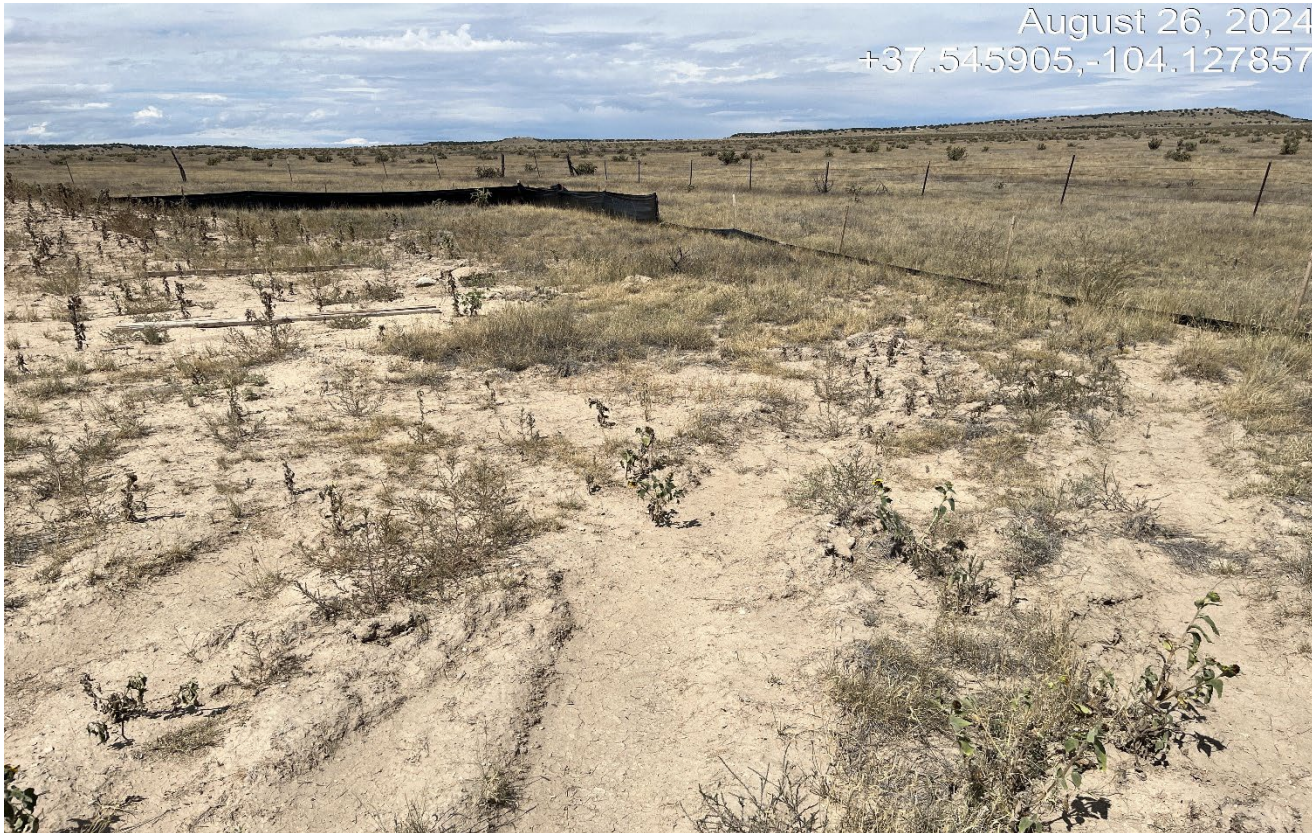
Photo 7. Facing toward the west corner of the location. The silt fence still remain down in this area.
