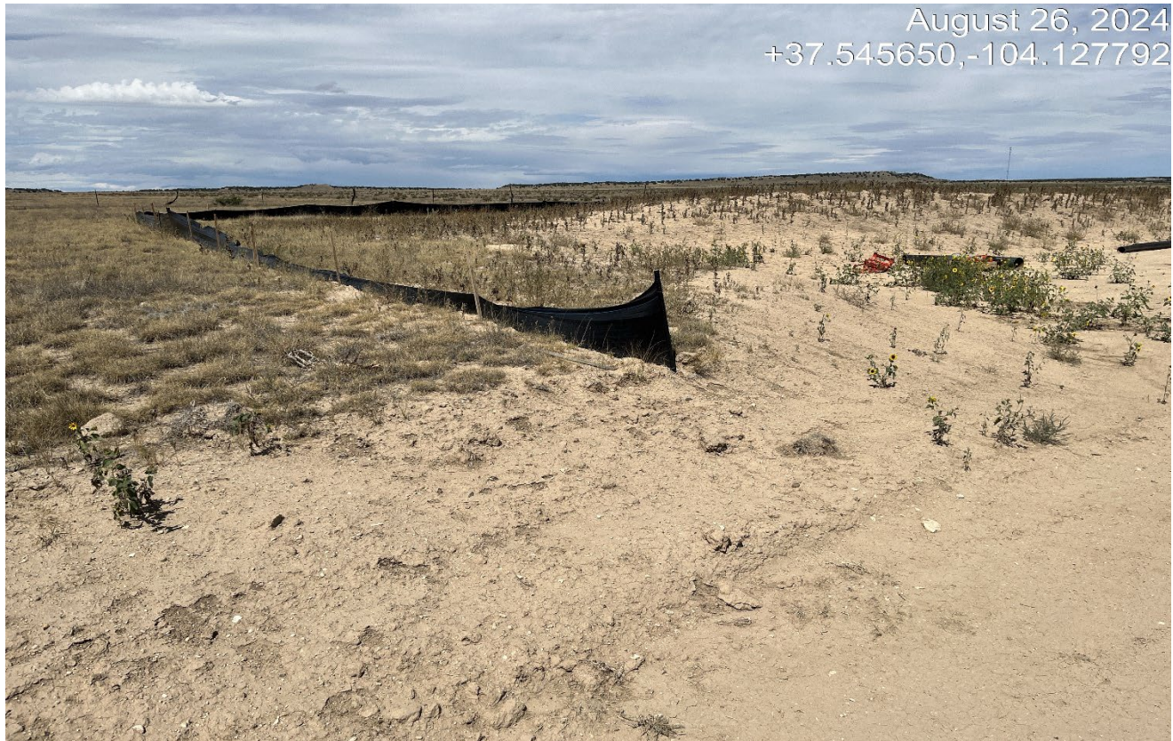
Photo 5. Facing southwest at the location. The silt fence is not maintained.
