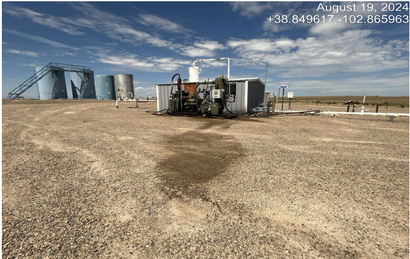
Photo 4. There is oil stained soils that has spilled out from the engine skid. The stained soils must be cleaned up and properly disposed.
