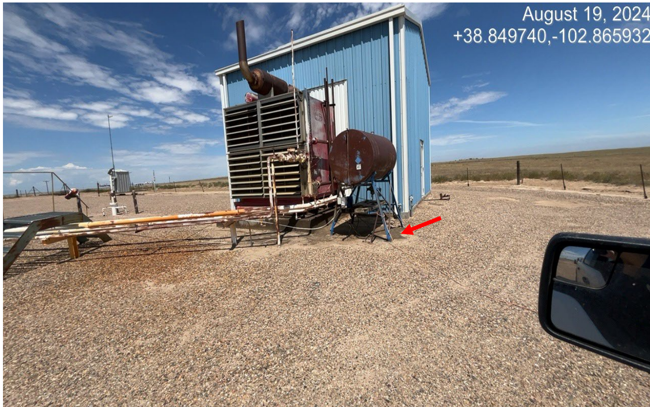
Photo 6. The fuel tank has leaked and has no secondary containment. Stained soils must be cleaned up and properly disposed.
