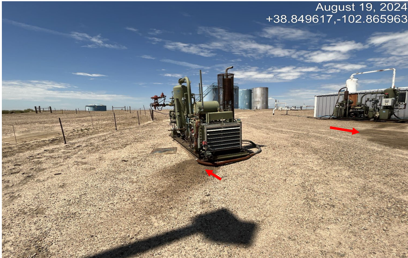
Photo 5. There is stained soils around the engine that needs to be cleaned up. The engine on the left appears to be unused and must be removed. The stained soils must be cleaned up and properly disposed.
