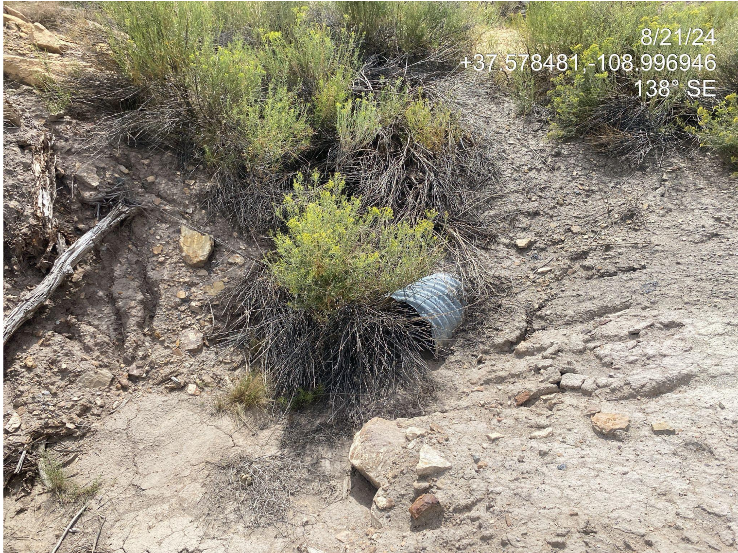
Photo 5. Culvert at access point is starting to fill with sediment, future maintenance is advised.
