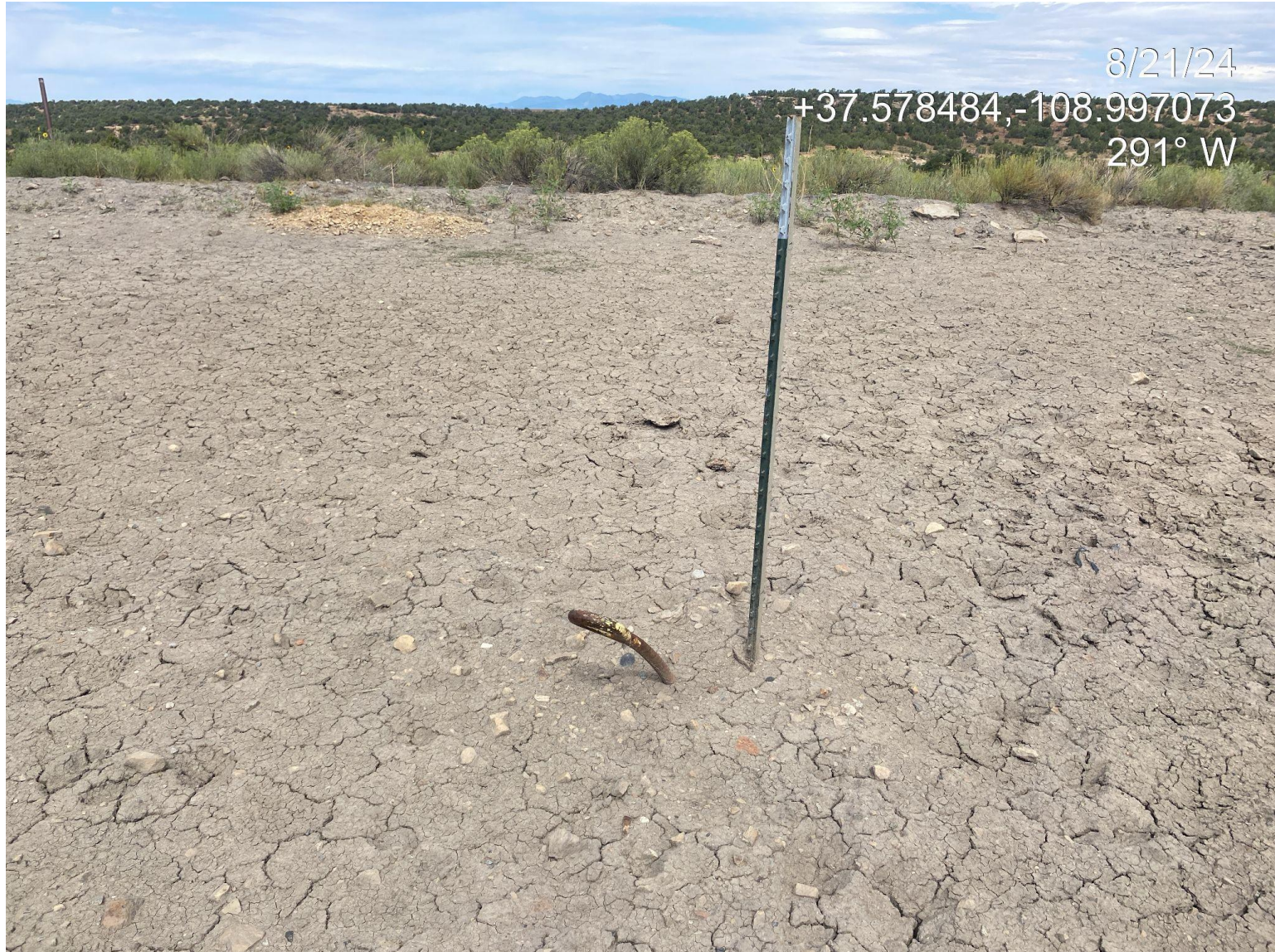
Photo 3. Guy line anchors on location have been properly marked.
