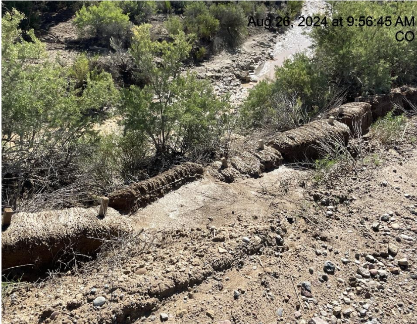
Photo # 6375 Hay bales/BMP's near creek/drainage have a large amount of sediment buildup & may need maintenance in the near future.
