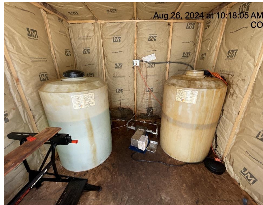
Photo # 6374 Chemical tanks in shed lack BMP's
