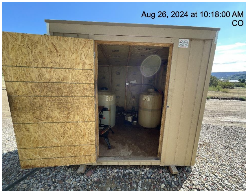
Photo # 6373 Chemical tanks in shed lack BMP's
