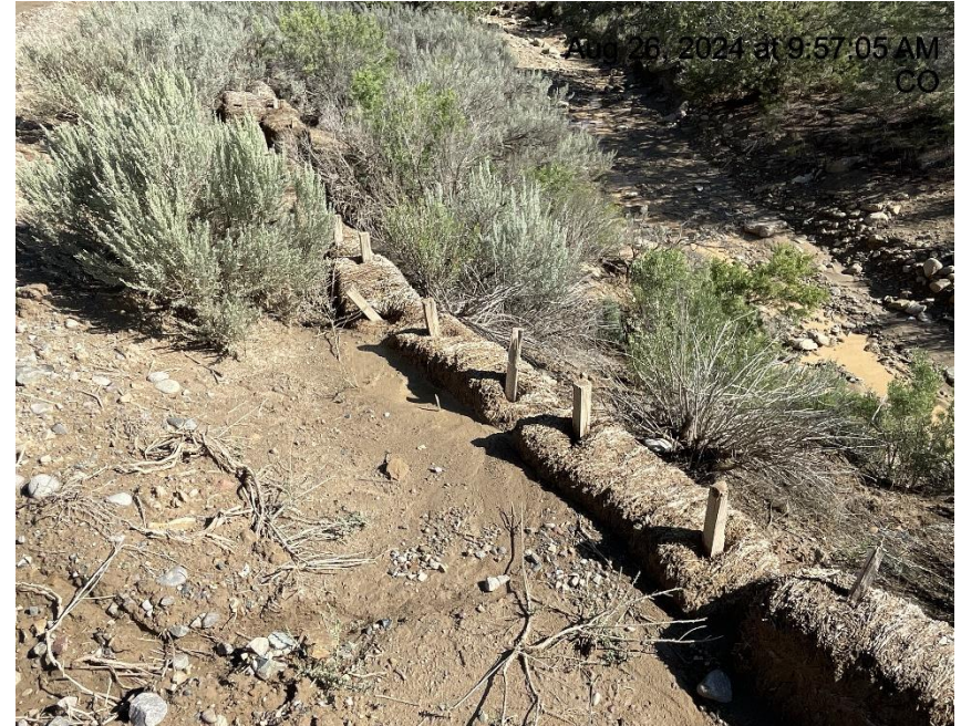
Photo # 6376 Hay bales/BMP's near creek/drainage have a large amount of sediment buildup & may need maintenance in the near future.
