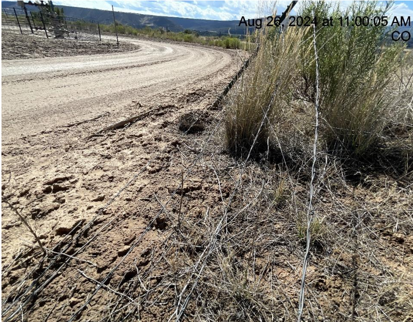
Photo # 6552 Barbed wire fence needs maintenance/wildlife hazard
