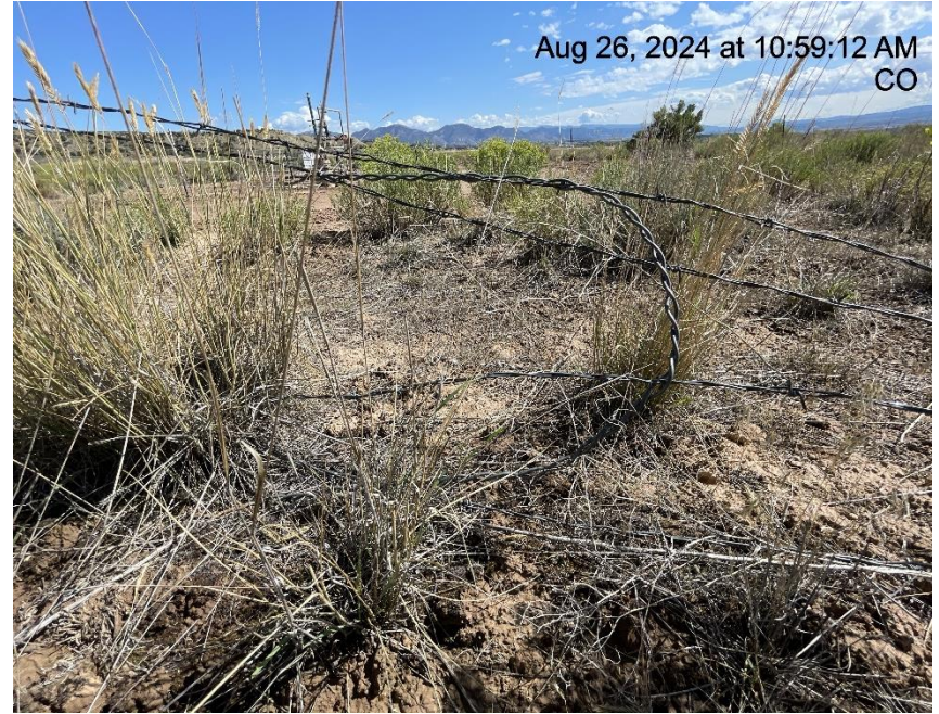
Photo # 6549 Barbed wire fence needs maintenance/wildlife hazard
