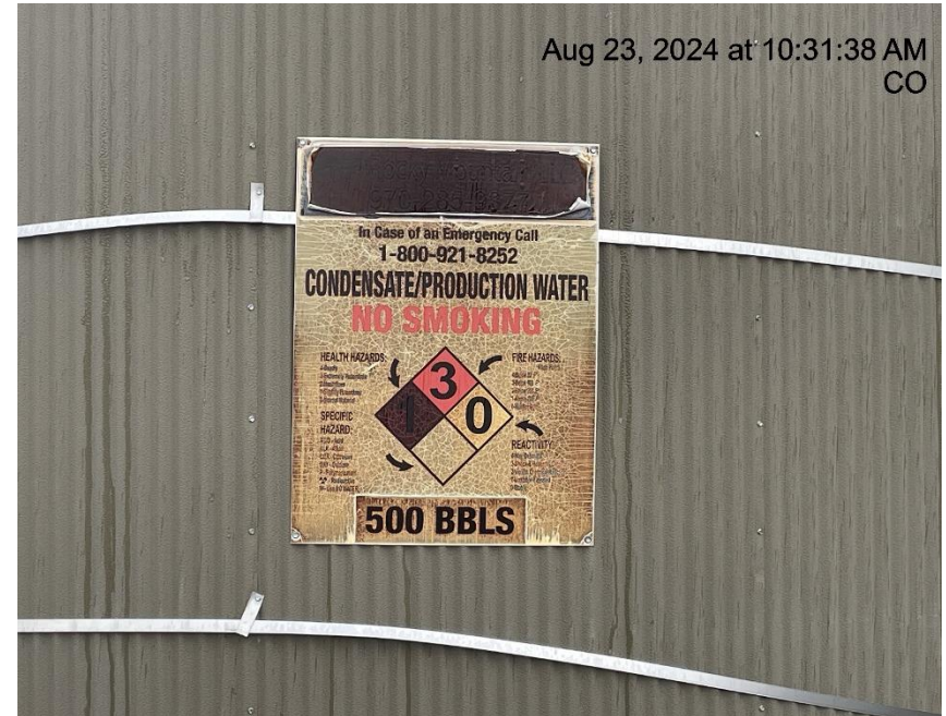
Photo # 6063 Tank label weathered & some required info is illegible/does not comply with CECMC labeling rules
