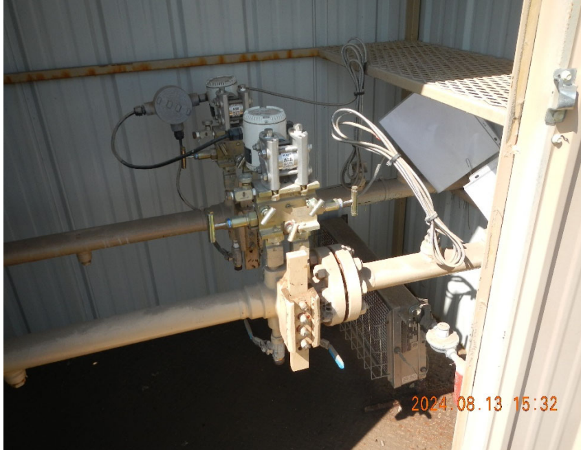
5. Digital gas meter inside remote meter shed.
