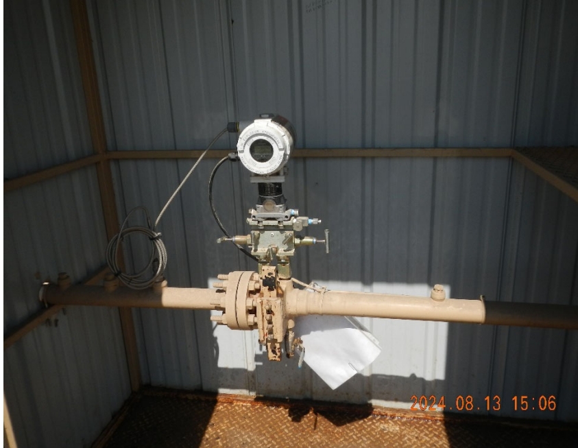
3. Digital gas meter inside meter shed.
