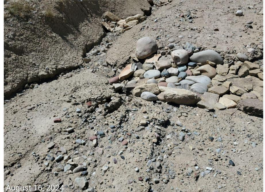
**Photo 1:** An armored outlet has been implemented on the east end of the Location. Controls to properly divert stormwater to the outlet do not appear to have been implemented in conjunction with the outlet. Stormwater scouring/degradation is becoming evident at sides of the BMP.
