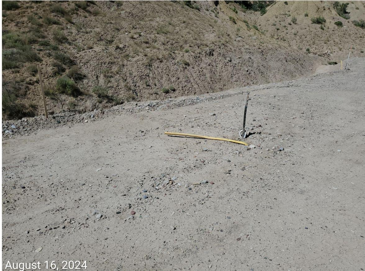
**Photo 2:** Marker at anchor has not been maintained and/or does not comport with 603.j requirements.
