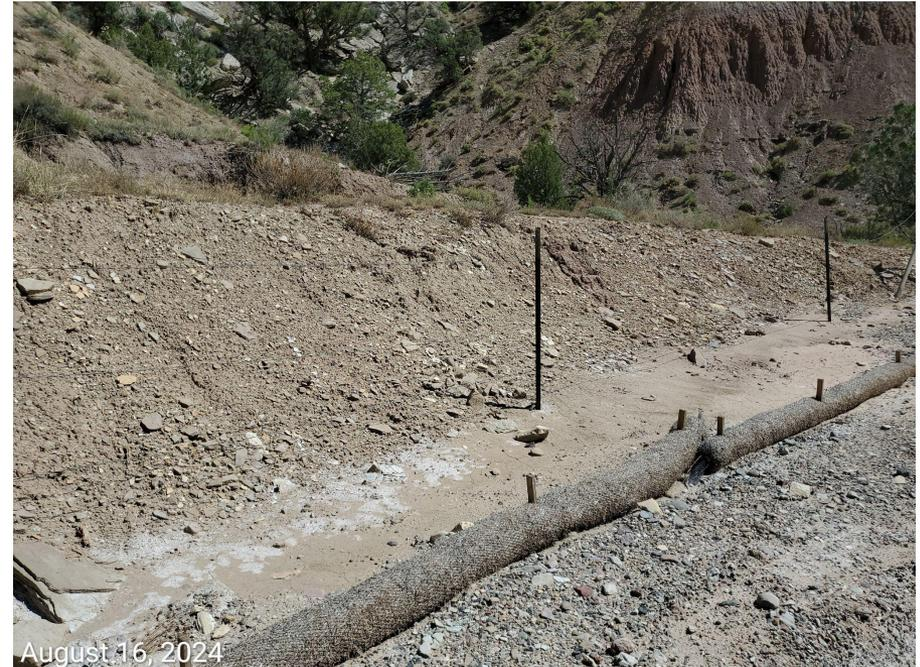
**Photo 2:** BMPs to stabilize, as well as to minimize erosion and degradation remain missing or insufficient at the slopes on Location. Lighter soils at toe of slopes sediment deposition due to unstablized slopes.
