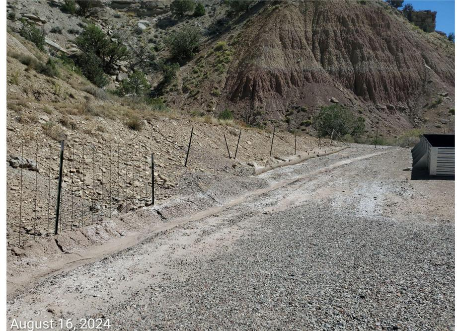
**Photo 1:** BMPs to stabilize, as well as to minimize erosion and degradation remain missing or insufficient at the slopes on Location.
