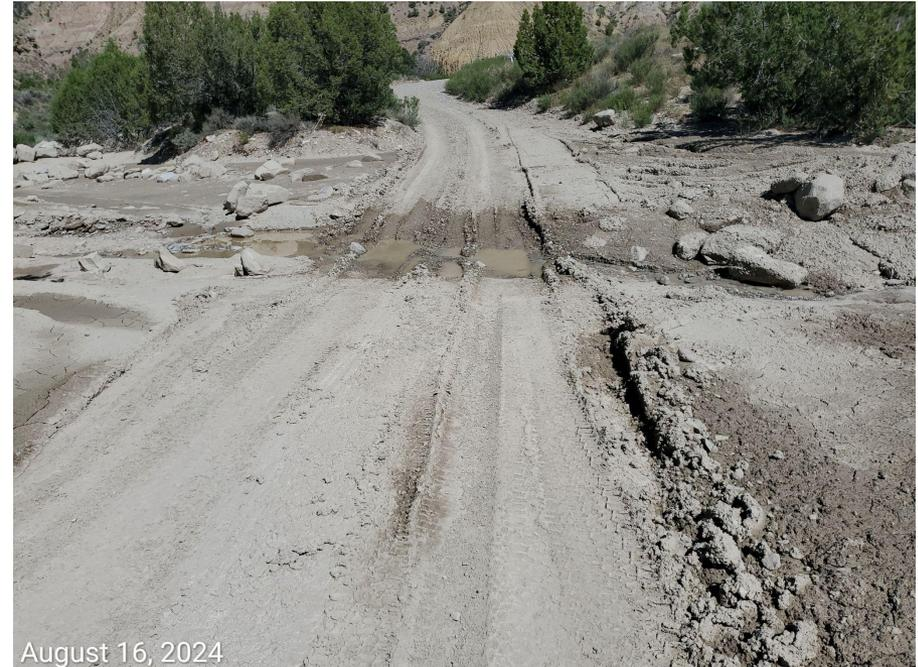
**Photo 1:** Photos 1-3 taken from the access road. Photos show BMPs, including a properly engineered stream crossing, has not been installed or maintained at the access road; degradation has persisted at the stream crossing.
