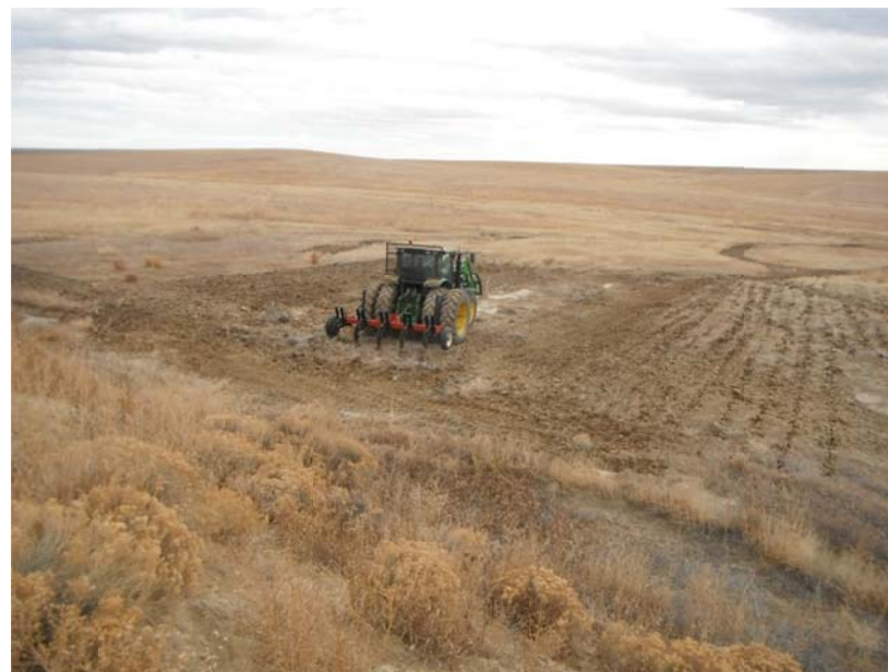
Deep ripping of impacted soils
