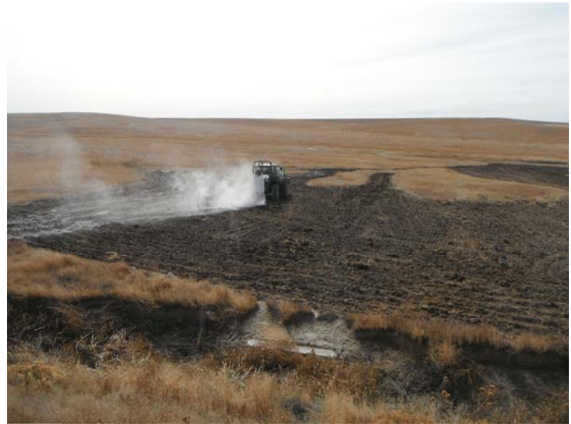
Application of solution grade gypsum
