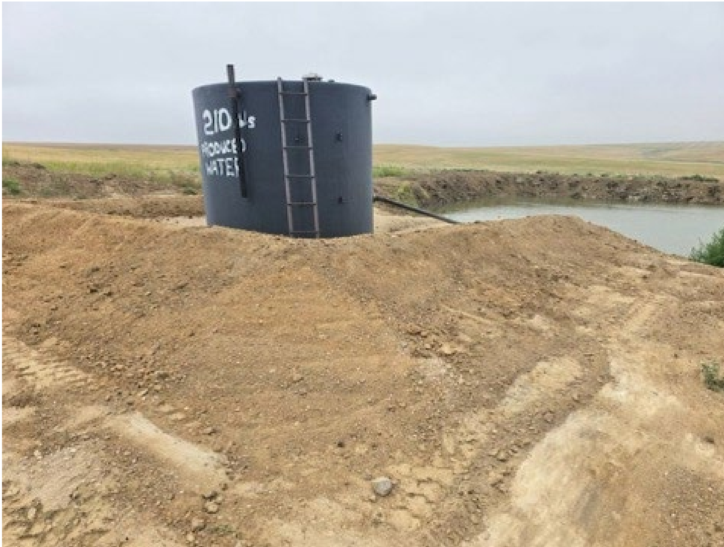
Repaired Berm around tank
