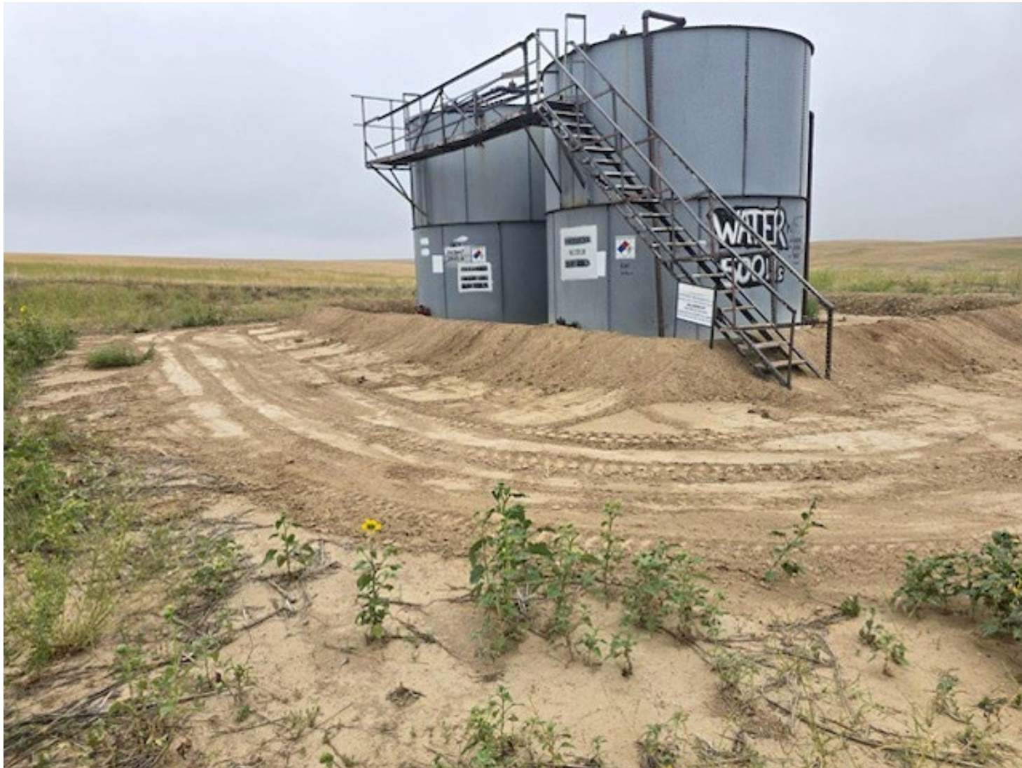
Repaired Berm around tank
