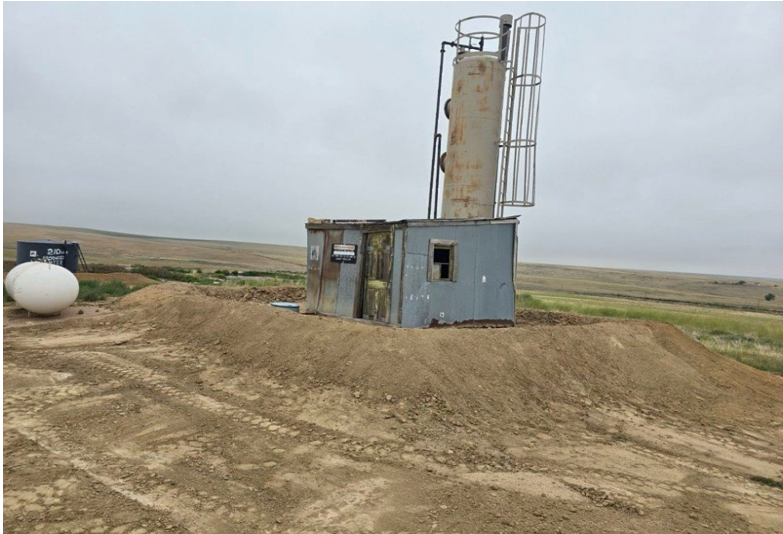
Repaired Berm around tank
