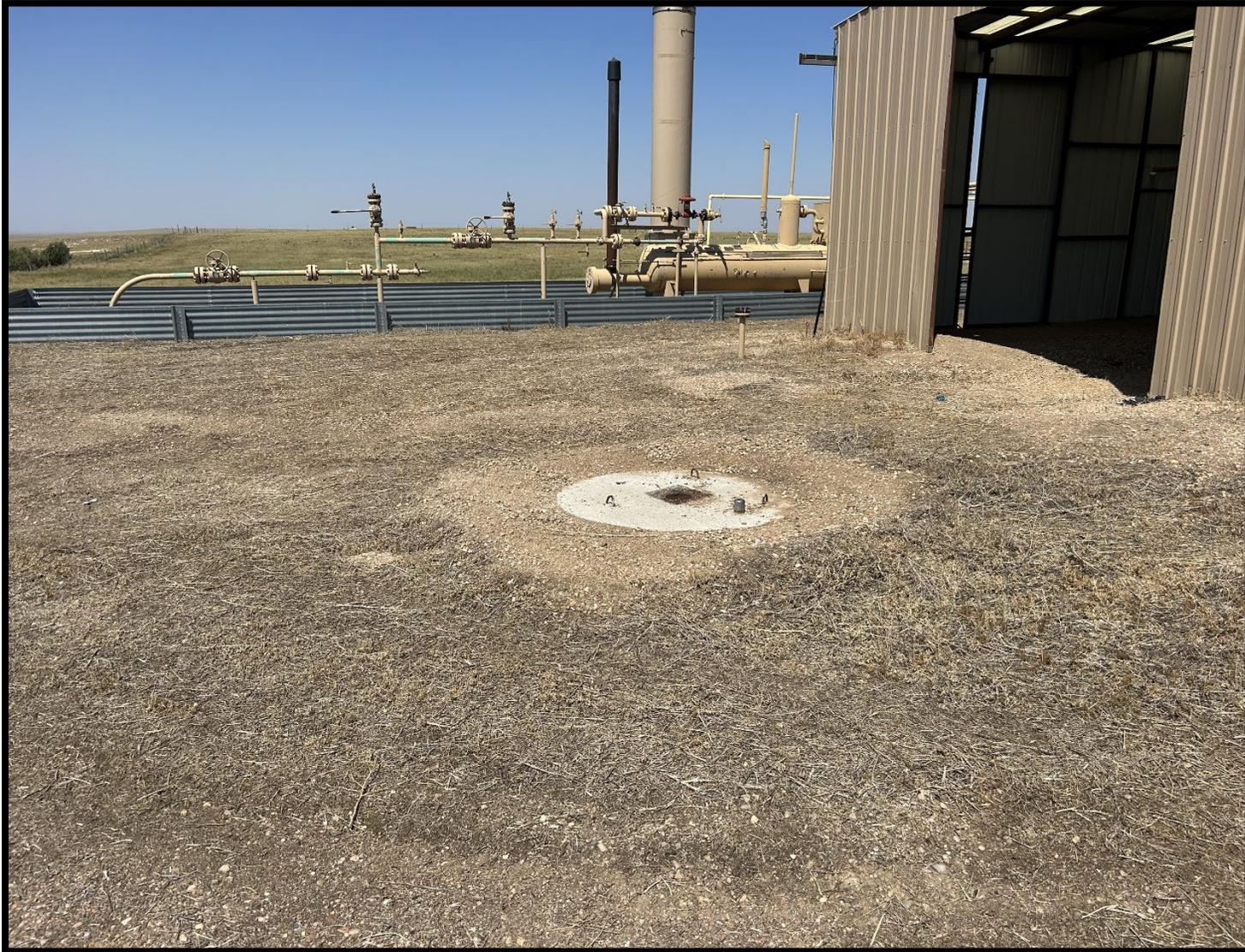
**CA:** Stained Soil at Compressor drain vault, see photos. For localized stained soils or oily waste - "Properly dispose of oily waste in accordance with 907.e."
