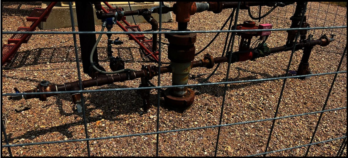
**CA:** Stained soil around wellhead. Comply with Rule 603.f.
