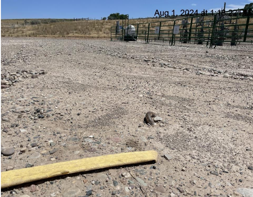
Photo # 4439 Improperly marked deadman
