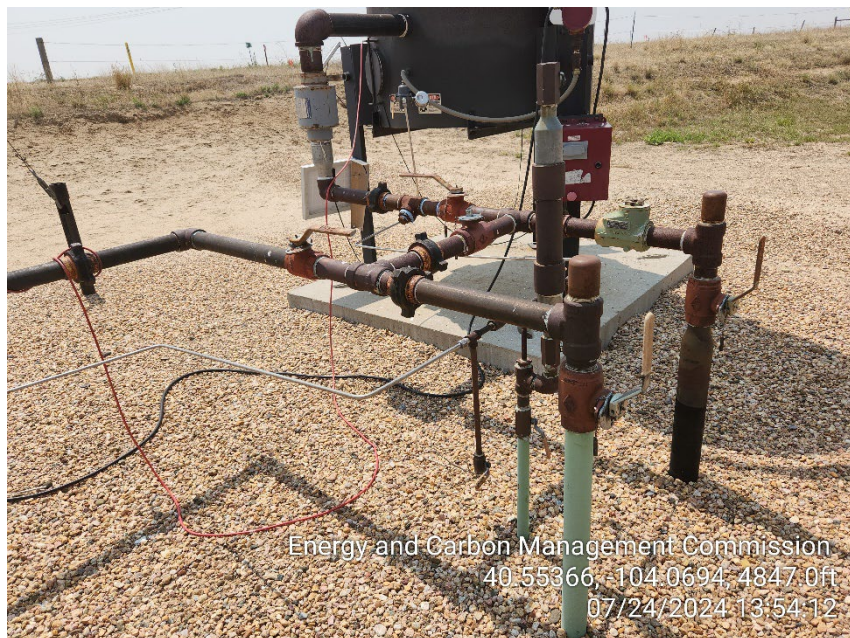
Photo 5 – Valves to Flare appear to be in Open position
