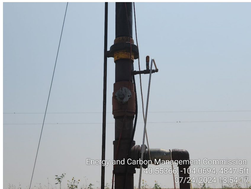
Photo 6 – Pilot Supply Valve appears to be in Closed position
