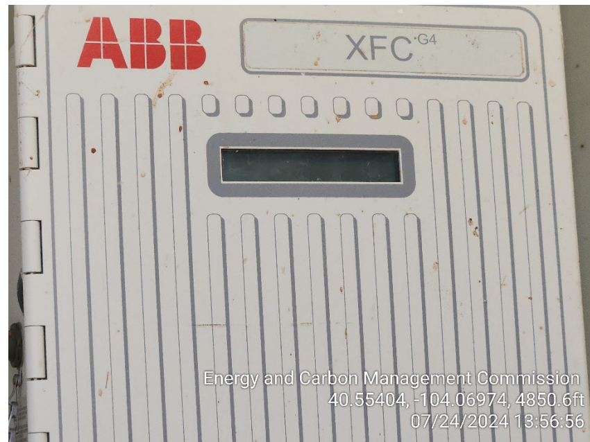
Photo 16 – Gas Sales Meter appears to be powered off
