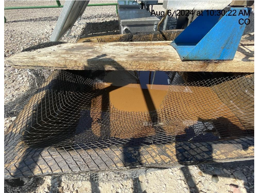
Photo # 4880 Netting/wildlife protection on containment needs maintenance/netting is sagging & partially submerged in unknown fluid/wildlife hazard
