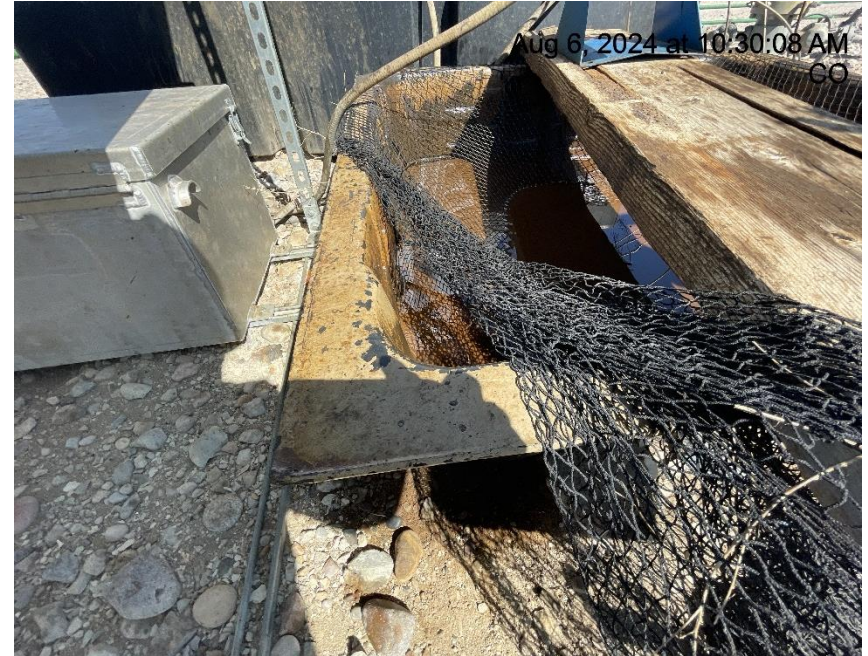
Photo # 4878 Netting/wildlife protection on containment needs maintenance/containment open to entry by wildlife /wildlife hazard
