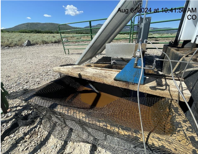
Photo # 4879 Netting/wildlife protection on containment needs maintenance/netting is sagging & partially submerged in unknown fluid/wildlife hazard
