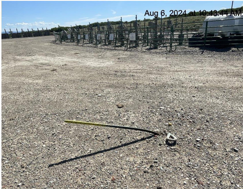
Photo # 4883 Improperly marked deadman
