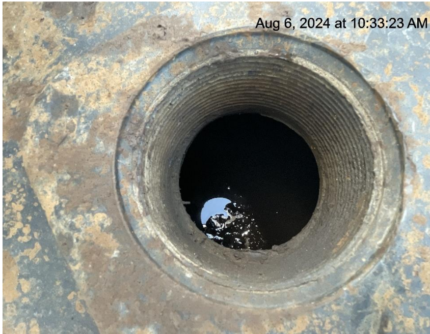
Photo # 4888 Failure to maintain chemical BMP - Chemical tank containment approximately 3/4 to 7/8 full of fluid/BMP insufficient to contain possible spill
