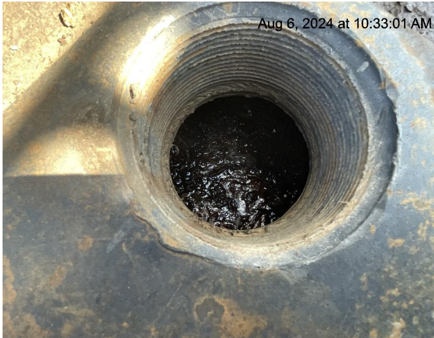
Photo # 4886 Failure to maintain chemical BMP - Chemical tank containment approximately 3/4 to 7/8 full of fluid/BMP insufficient to contain possible spill
