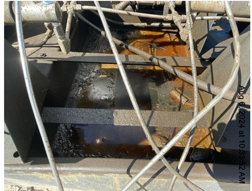
Photo # 4887 Standing fluid on top of chemical tank containment/wildlife hazard
