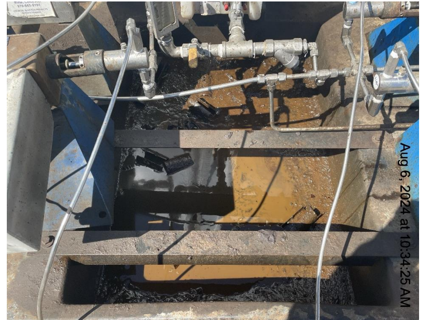
Photo # 4889 Standing fluid on top of chemical tank containment/wildlife hazard
