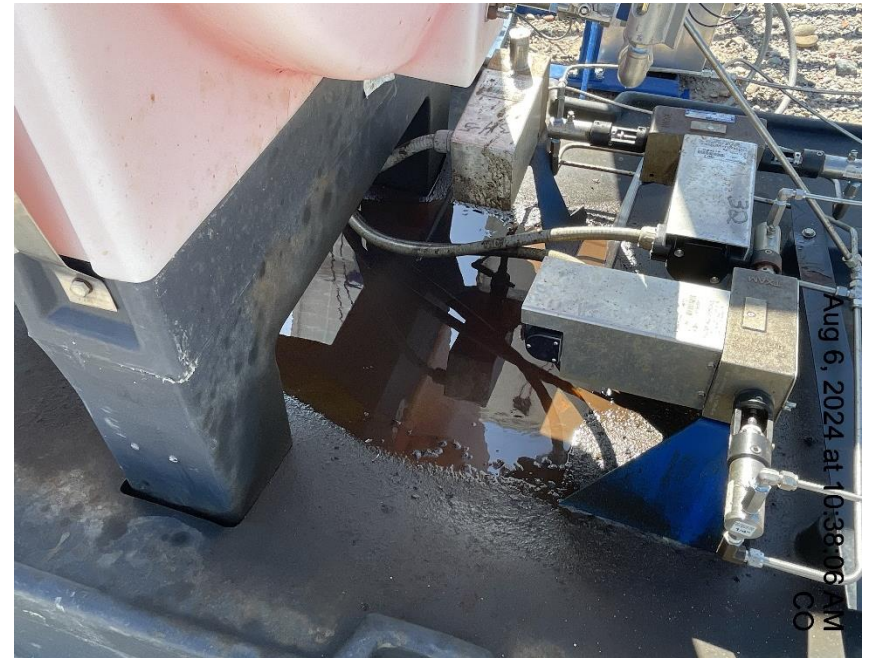
Photo # 4885 Standing fluid on top of chemical tank containment/wildlife hazard
